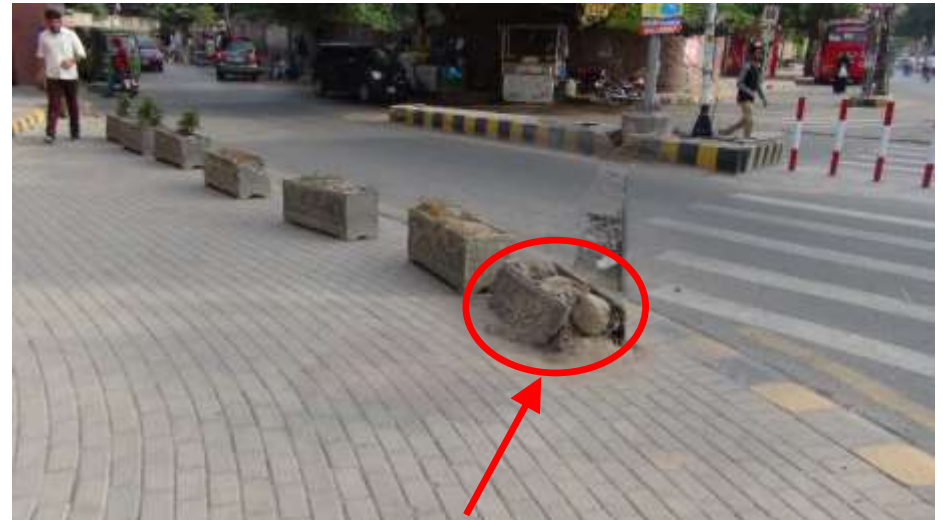
Some planters are already damaged
