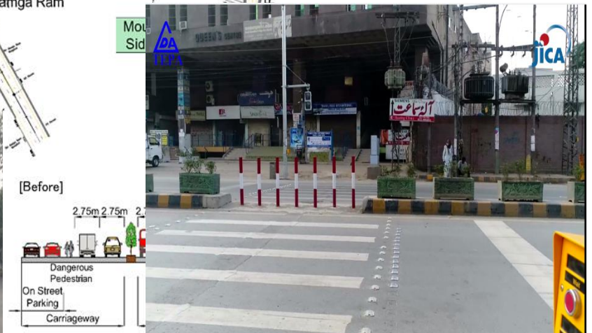
Pedestrian Crossing with Pelican Signal
