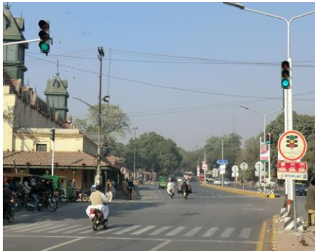
① Functioning traffic signal at Mall Road near Anarkali
