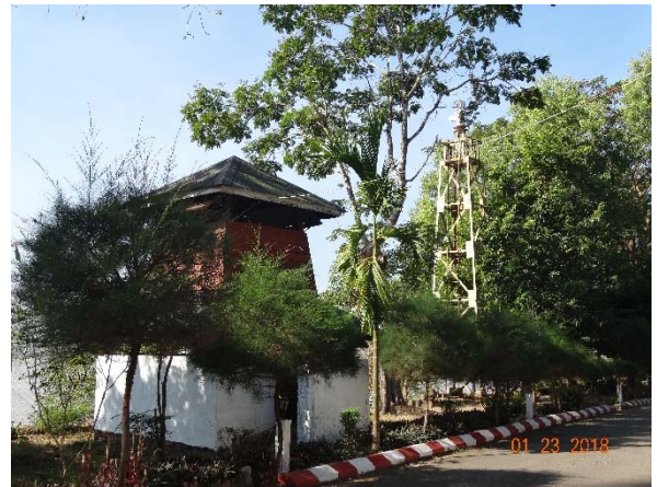
Photo: The Area near Existing Monkey Point Light Tower (In Navy Compound)
