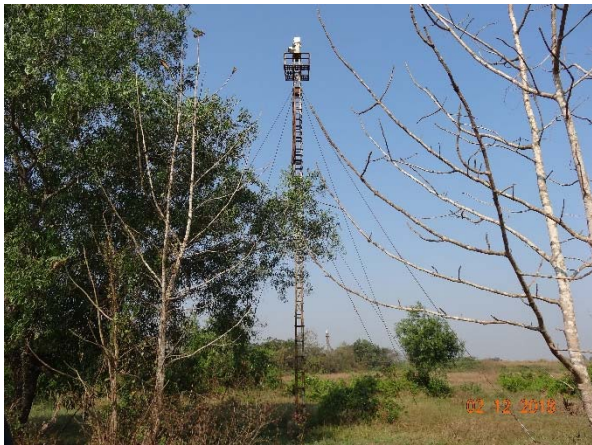
Photo: The Area near the Existing Thanlyin Point Light Towers
