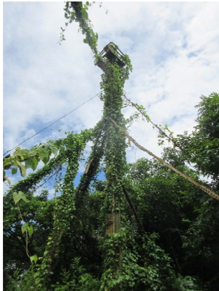
Photo: The Existing Thanlyin Point (Front) Light Tower
