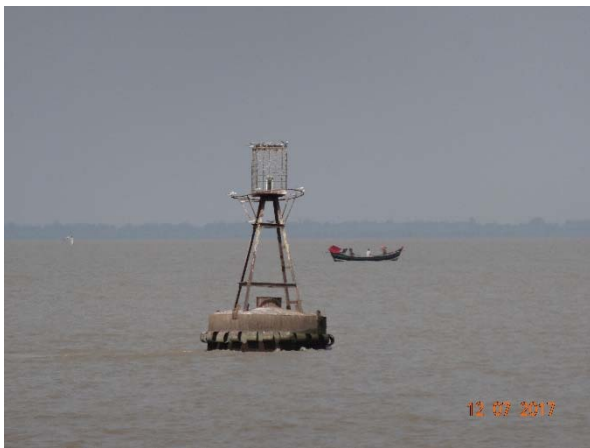
Photo: One of the Existing Navigation Buoy in Yangon River
