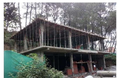
Under the Construction
