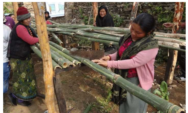
Hands-on training for construction of improved goat sheds
