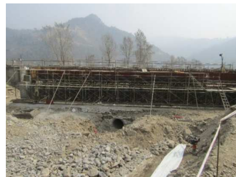
General View of Construction
