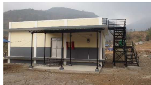
After completion photo of Seed Storage in Kiwool
