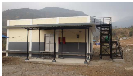
After completion photo of Seed Storage in Kiwool
