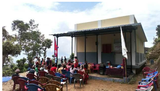
After completion photo of Seed Storage in Irkhu
