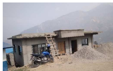
During the construction
