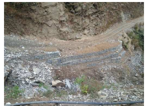
Gabion wall Construction
