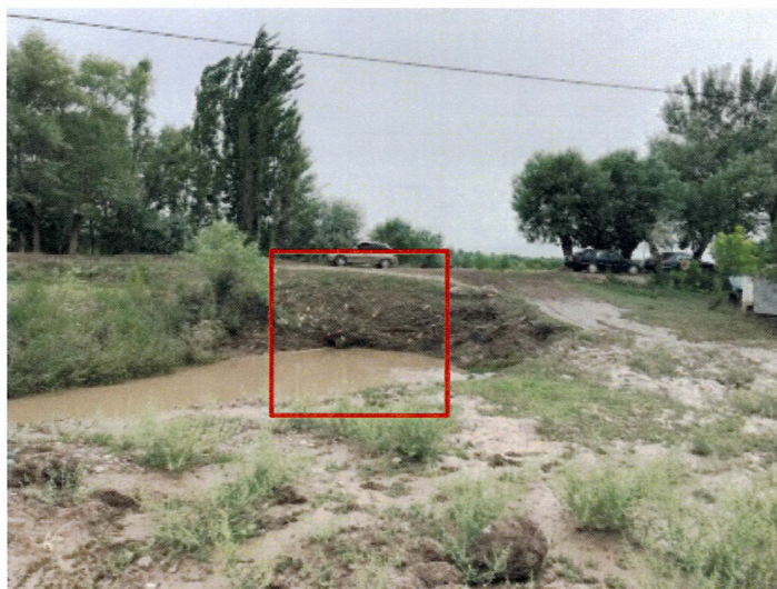
Figure-1. Existing Box Culvert
