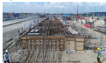
Figure 3.5.12 Concrete Work (Phase I)
