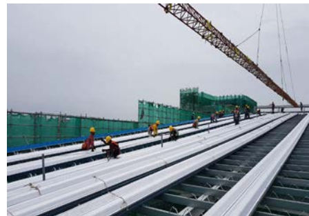
Figure 3.5.16 Steel Roofing Work (Phase I)
