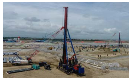
Figure 3.5.10 Piling Work (Phase I)
