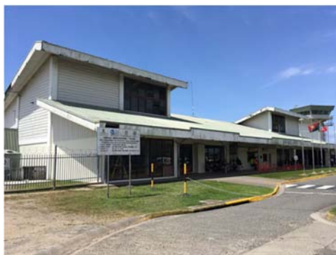
Photo 11 Exterior of Passenger Terminal
