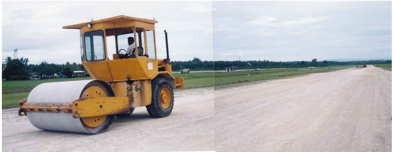
Photo 3 Runway Surface only Coral compacted (August 1995)
