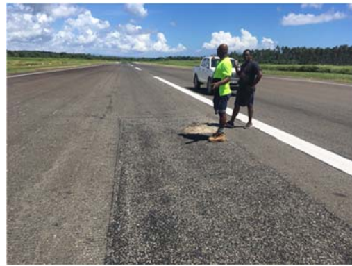
Photo 8 Repair of Runway Pavement (2)
