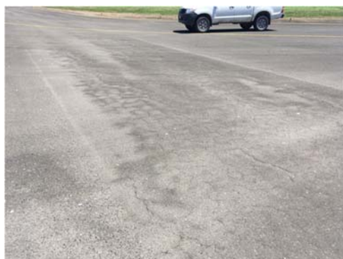
Photo 9 Condition of Runway Pavement (1)
