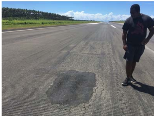
Photo 7 Repair of Runway Pavement (1)
