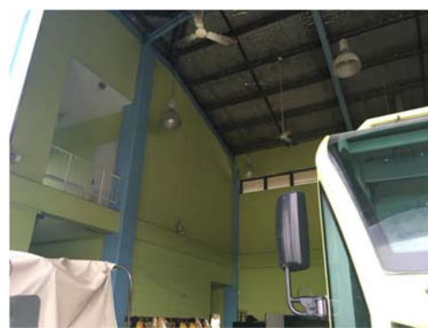
Photo 20 Interior Wall & Ceiling
