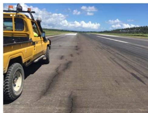
Photo 10 Condition of Runway Pavement (2)
