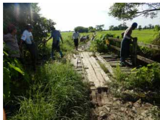
Figure 3-1-7 Timber decked bridge
