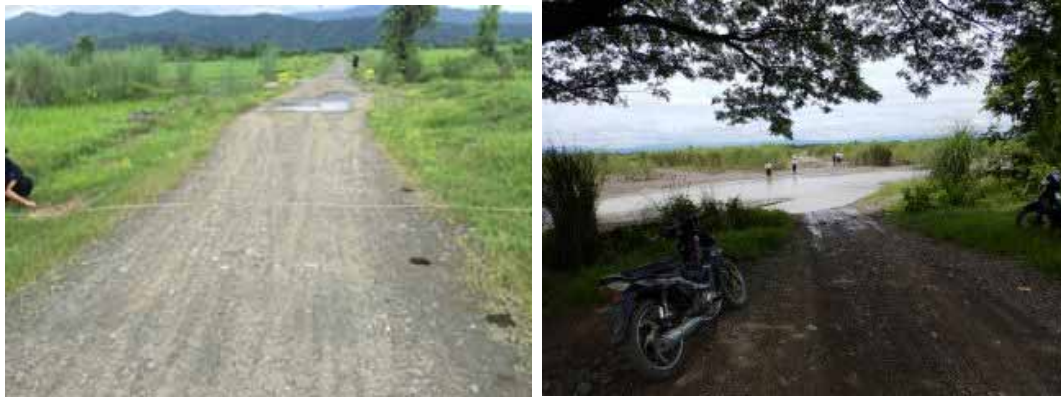
Figure 3-1-2 Current situation of Road A and planned bridge location
