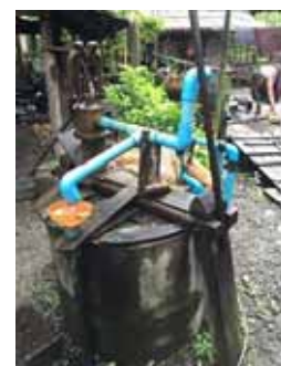
Existing shallow well in Zo Zang village
