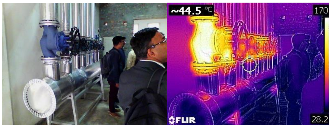
Figure 22 Thermal Image of Steam Valves of Header in Boiler Room
