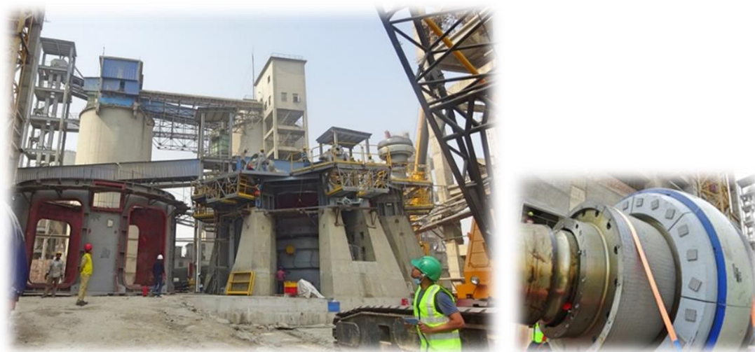
Figure 26 VRM and Grinding Roller under Installation
