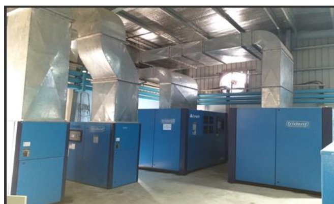
Figure 14 Photo of Installed Air Compressors
