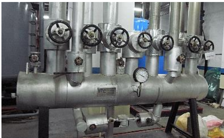
Figure 23 An example of insulation of steam valves
