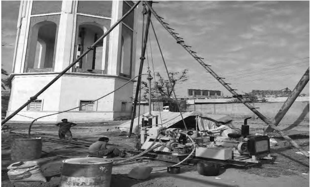
Boring in Progress at Abdullah Pur OHR
