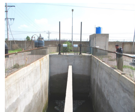
Inlet Channel and Inlet Gate
