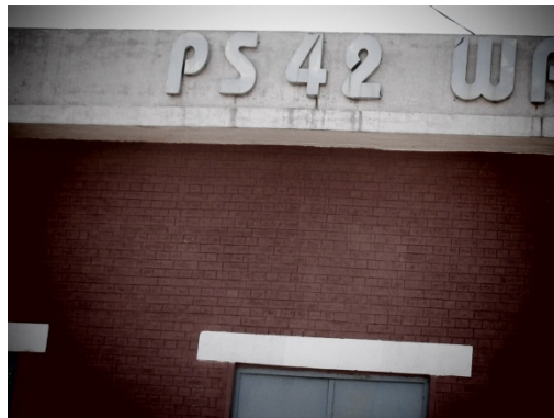
Name Plate at the Pump House
