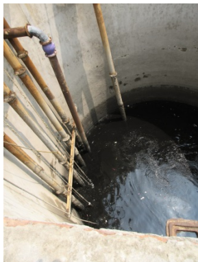
Receiving and Flow Adjustment Well
