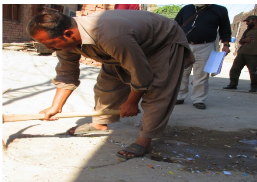
Investigation of Manhole Depth
