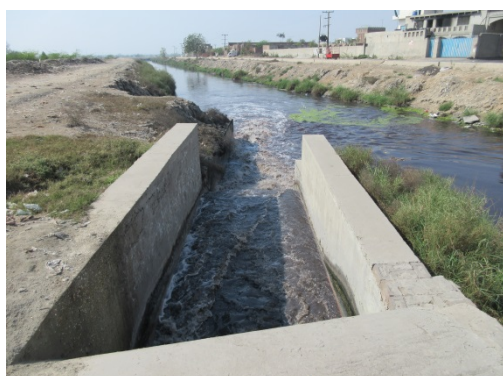
Discharge Point and Pharang Drain
