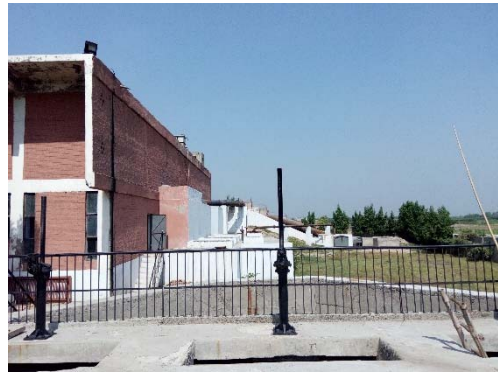
Overview from Inlet Chamber
