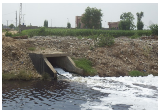
Discharge Point of Pharang Drain
