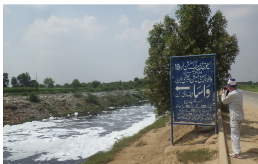
Discharge Point – Pharang Drain
