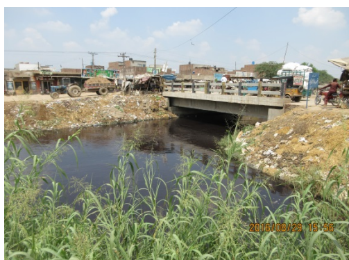
Discharge Point of Pahrang Drain
