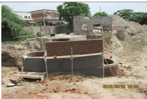
Under Construction of New Inlet Work
