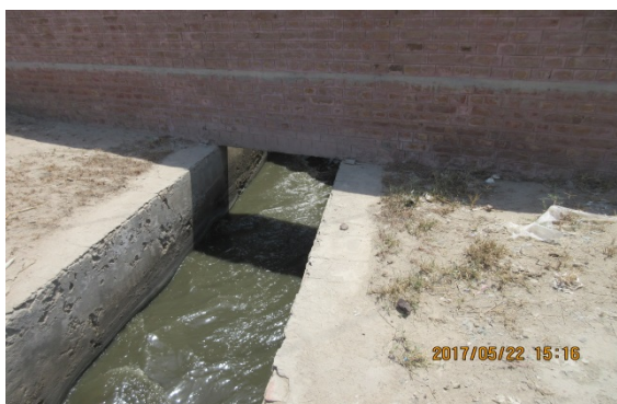
Discharge Channel to Dijikot Drain
