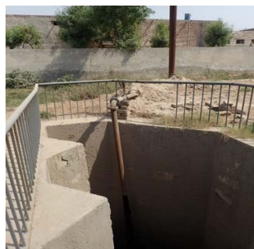
Preliminary Treatment Facility
