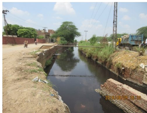
Discharge Pipe and Drainage Channel No.1
