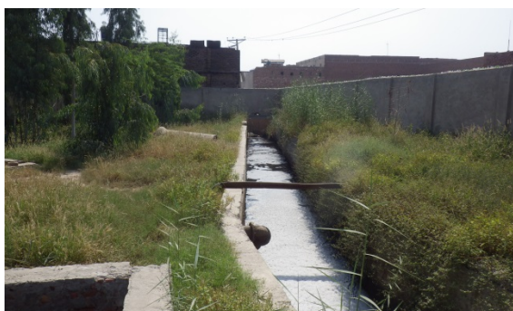
Receiving and Flow Adjustment Well
