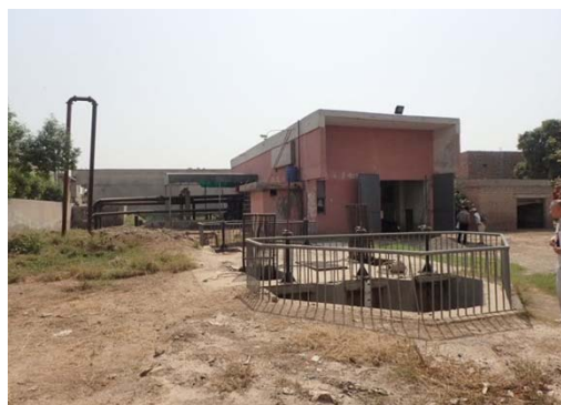
Inlet Work and Pump House
