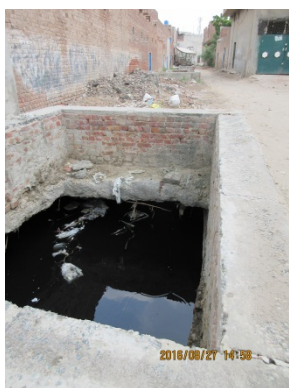
Drainage Point of Drainage Channel No.1g
