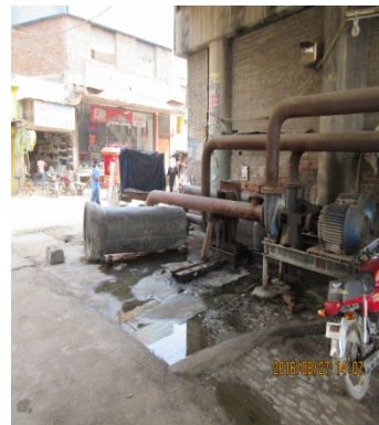
Pump Well and Equipment
