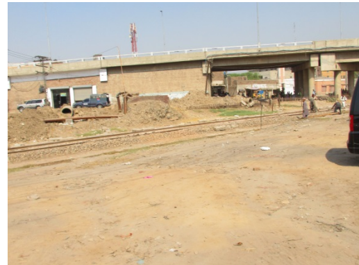
Overview of Delivery Chamber
