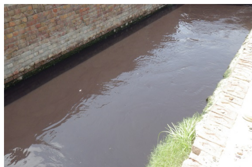
Satiana Road Sullage Drain
