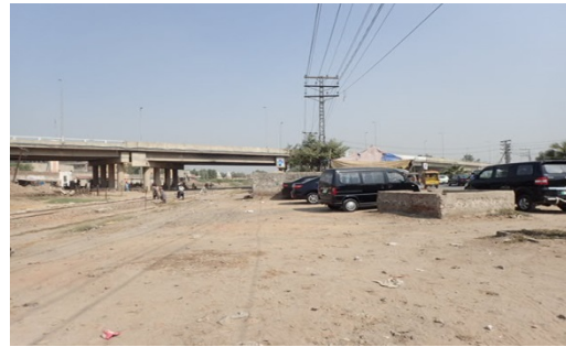
Overview of Inlet Chamber
