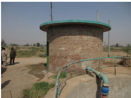
Pump House and Suction Pipe
