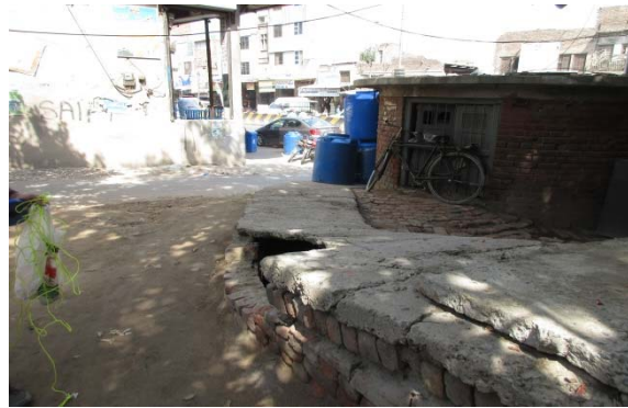
Discharge Channel goes to Sewer Pipe
