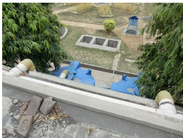
Pipe, tanks and concrete pits
