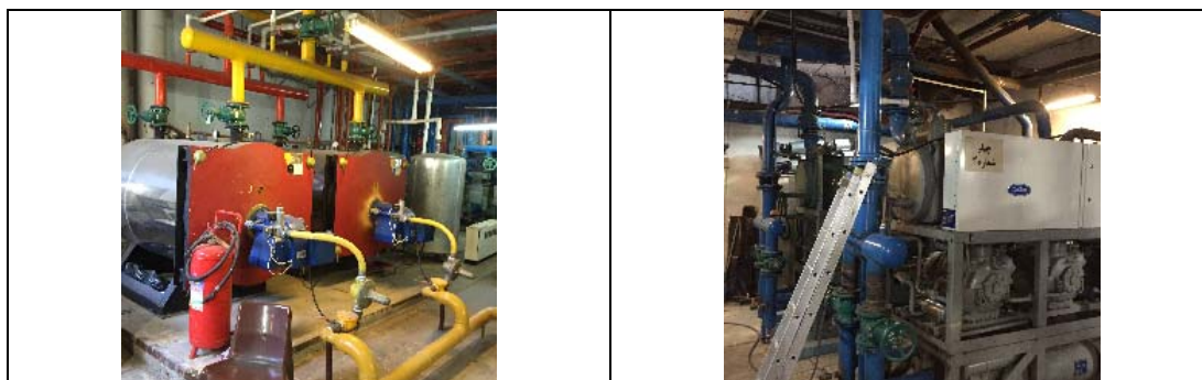
Source: Prepared by the JICA Project Team
