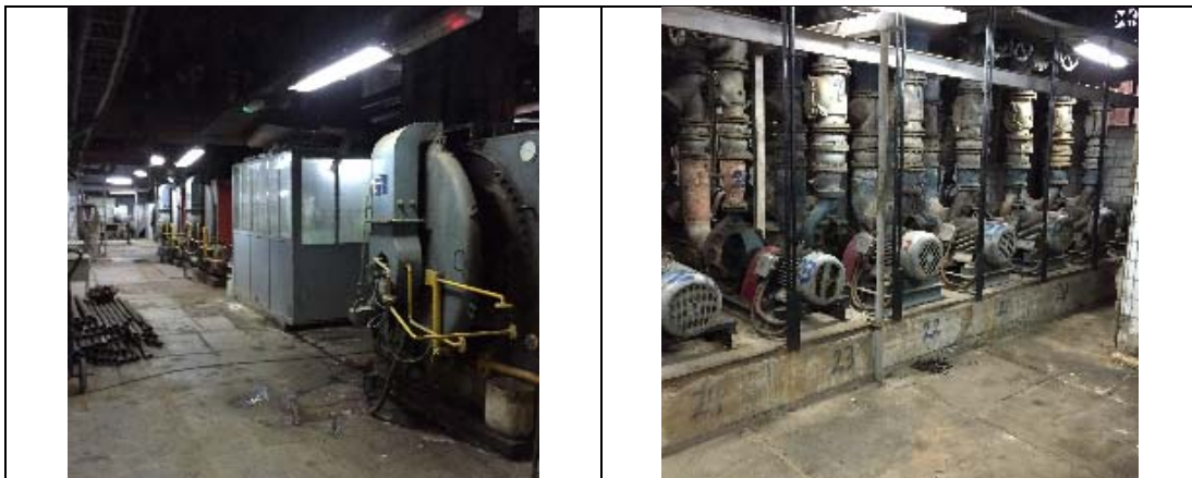
Source: Prepared by the JICA Project Team
