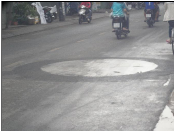
Steel Casing Shaft (Passing Shaft/Covering Plate are installed)
