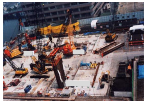
Figure 8.8-1 Underground Continuous Wall Construction Method (Reference Drawing)
