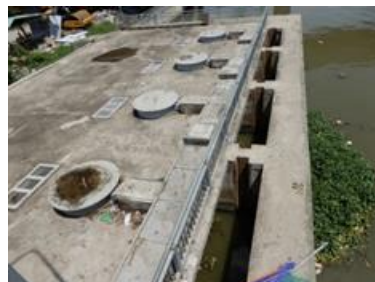
Installed four pumps at the right bank
