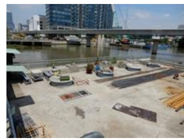
Installed four pumps at the left bank
