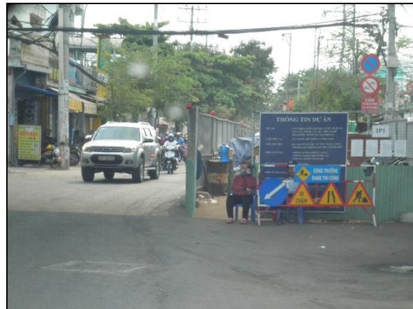
Steel Sheet Pile Shaft (Drive Shaft)
