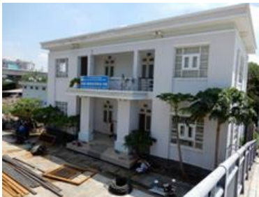
Main Tidal Control Gate Office
