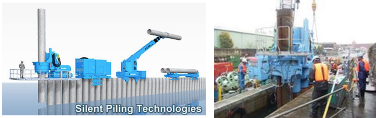
Figure 8.8-3 Steel Pipe Piling Method (Reference Drawing)
