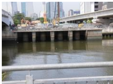
Inlet of four pumps on the right bank
