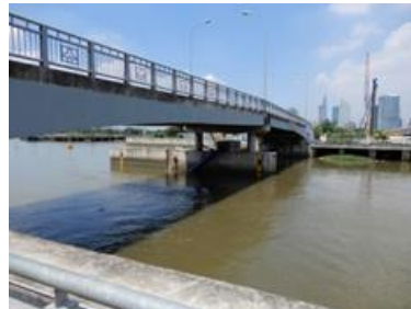
Tidal Control Gate on the left bank
