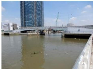
Panorama view of the Tidal Control Gate from Downstream
