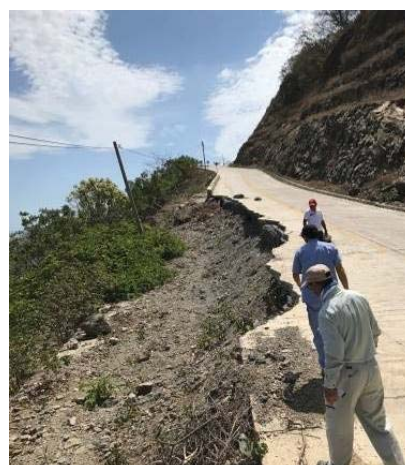
Picture 1: Road collaption site due to debris fall in rainy season in Carimbala area on National Road No.3
