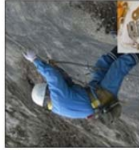
Safe Slope Work
