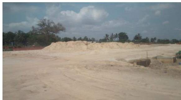
Photo 2-2 Ongoing Earthworks (Culverts on right hand side foreground) [MSBR]
