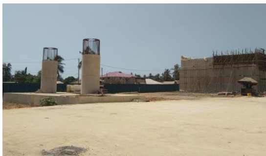
Photo 2-1 Kibundani Interchange (Adjoining to existing highway) [MSBR]
