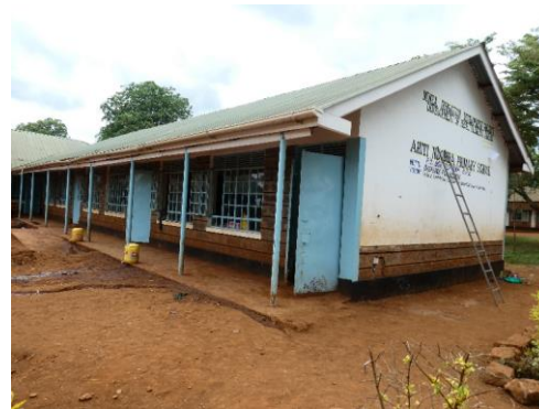
Photo 2-8 Renovated elementary school at the relocated site (Mwea)
