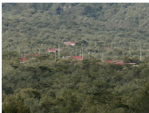
Photo 2-9 Housing complex at the relocation site (Olkaria)
