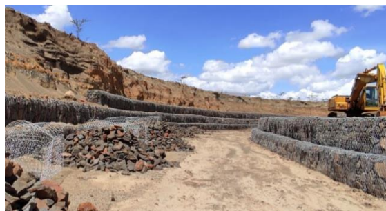
Photo 2-6 Inspection of Ongoing Protection Works in a Gully Crossing through Naivasha SEZ Land
