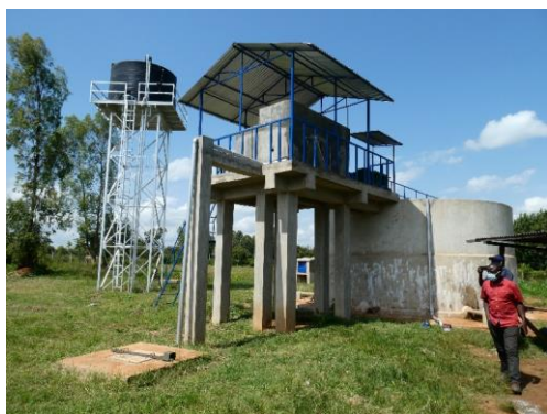
Photo 2-7 Water supply facilities at the relocation site (Mwea)
