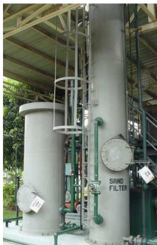
Figure 6 Valveless Sand and Activated Carbon Filters and Effluent of Activated Carbon Filter
