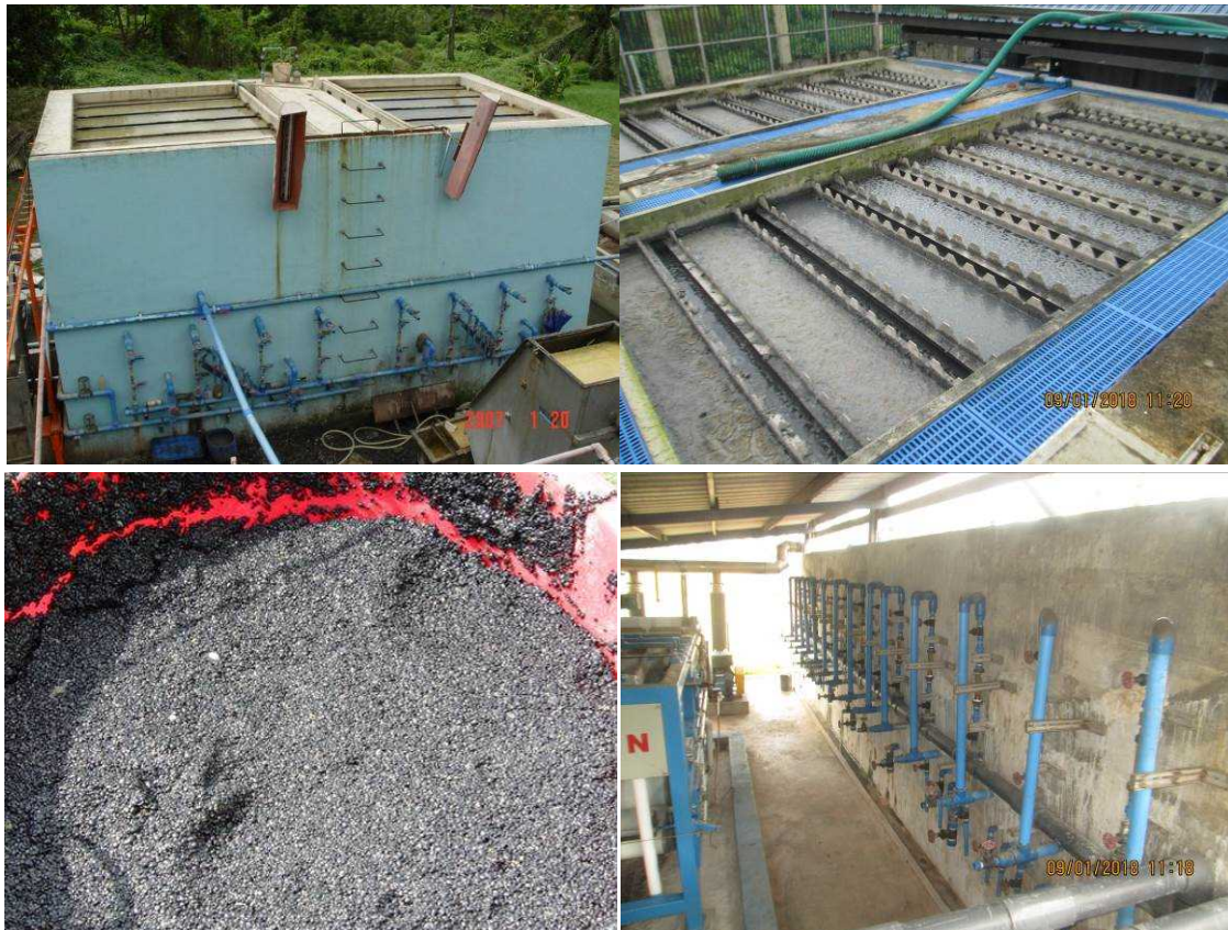
Figure 14 Upflow Anaerobic Sludge Blanket (UASB) Reactor, Overflow / Effluent Collection Channels, Bottom Feed Flow Control System, and UASB Granules (clockwise from top left)
