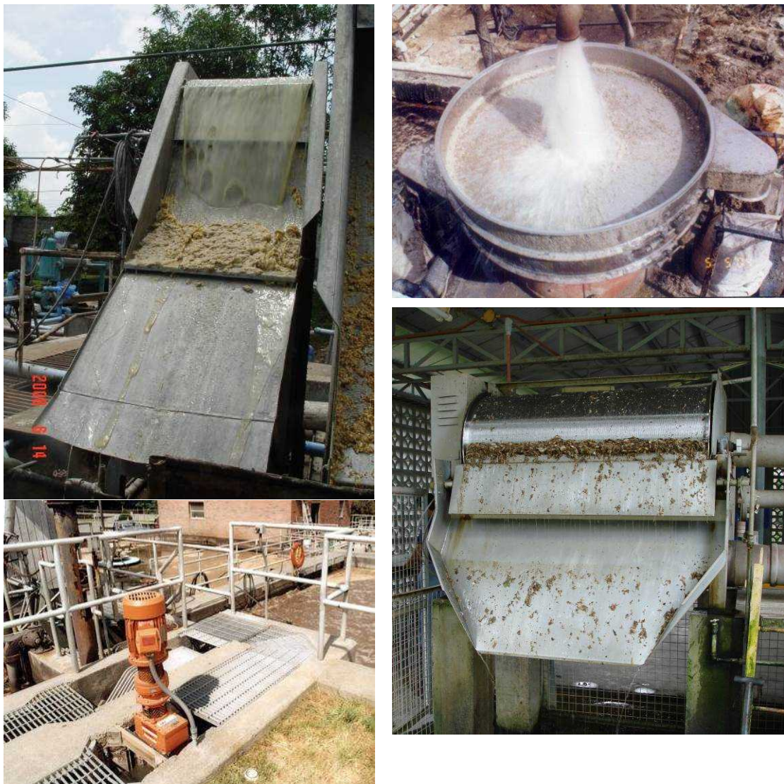
Figure 1 Examples of Static Screen, Vibratory Screen, Rotary Drum Screen, and Comminutor (clockwise from top left)
