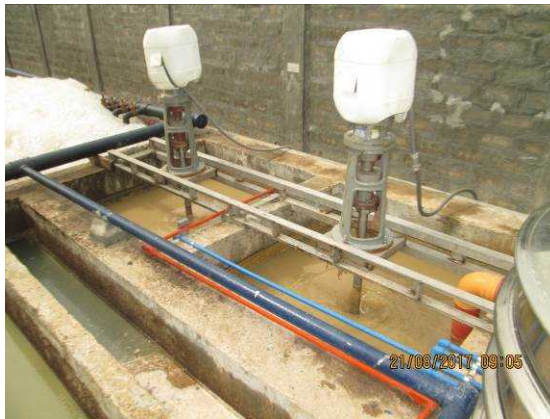
Figure 8 Examples of Flash Mixing and Flocculation Units
