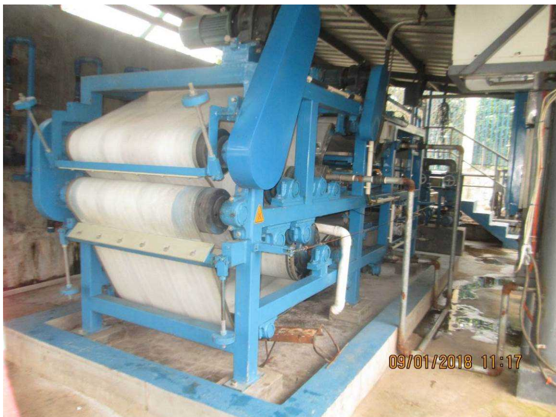
Figure 18 Belt Filter Press
