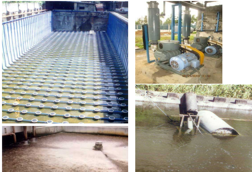
Figure 11 Aeration Systems: Diffused Aeration with Blowers, Aspirating Mechanical Aerators, and Conventional Mechanical Surface Aerators (clockwise from top left)
