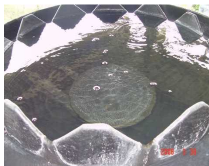
Figure 6 Valveless Sand and Activated Carbon Filters and Effluent of Activated Carbon Filter
