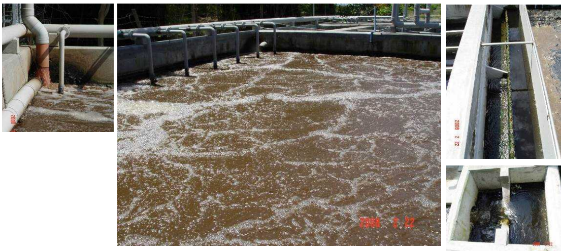
Figure 10 Activated Sludge Treatment Plant: Influent, Aeration Tank, Effluent Launder (Channel), and Flow Metering Effluent Weir Box
