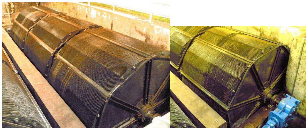
Figure 13 Rotating Biological Contactors (RBC) with Mechanical Drive
