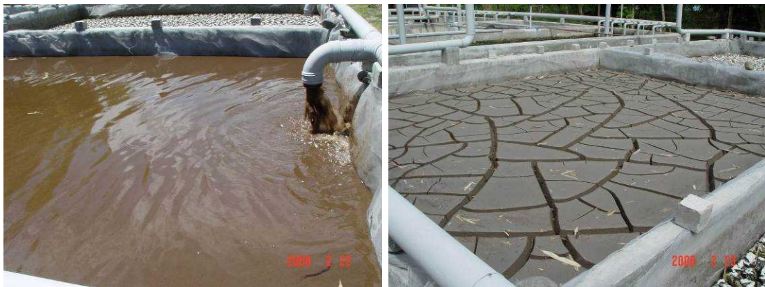
Figure 16 Filling Sludge Drying Bed and Dewatered / Dried (Waste Activated) Sludge
