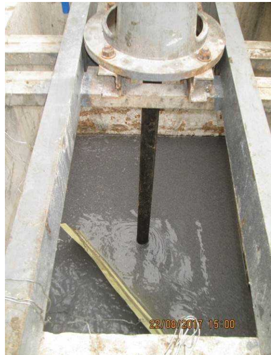
Figure 8 Examples of Flash Mixing and Flocculation Units
