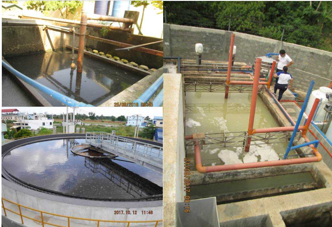
Figure 4 Examples of Sedimentation or Settling Tanks or Clarifier
