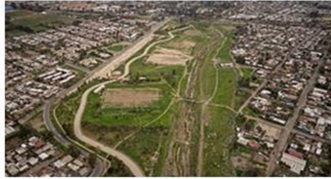
Macul ravine and the park of the same name, built in the construction exclusion zone.
