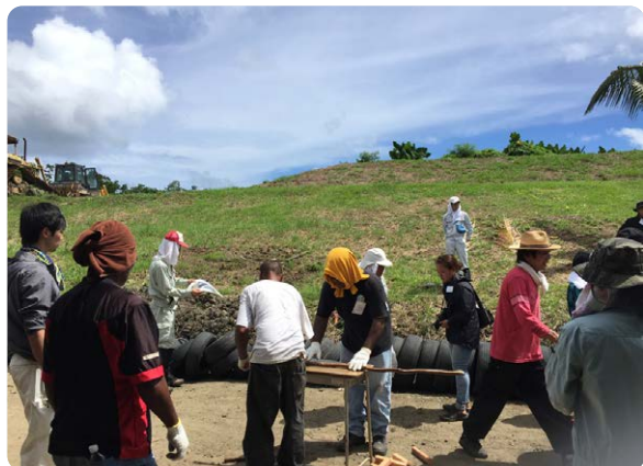
Demonstrating how to make a drainage pipe from used tires (2018)
