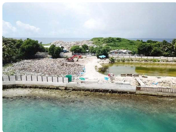
Extension to the lagoon-side (2021)
