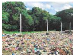
Vertically extended landfill gas venting pipes
