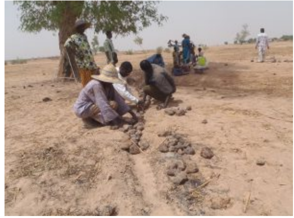
Construction of stone barriers
