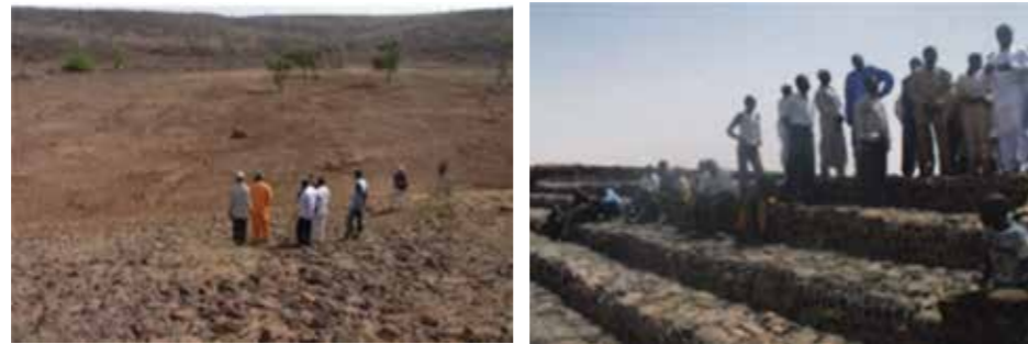
A water reservoir whose water has run out during the dry season A water reservoir repaired in Bakassomouba
