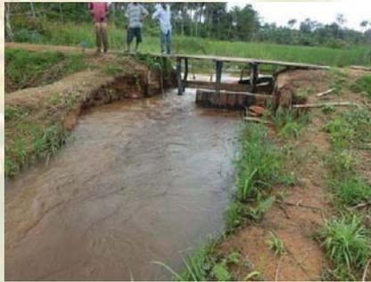
Spillway destroyed by a flood(29/8/2019)
