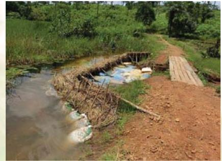
Simple weir constructed to check water(18/9/2019)
