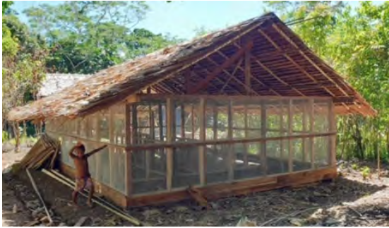
Chicken shed (Komuniboli) under construction (May 2022)
