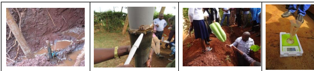
Figure-11 Overview of Verification work by Excavation
