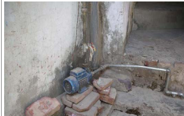
(2) Booster pumps in service line
