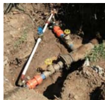
Bypass line & Flow meter
