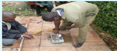
Connect pump with pipe and place water pressure
