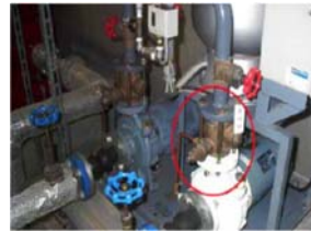
Install a reducing valve in the pump discharge side.
