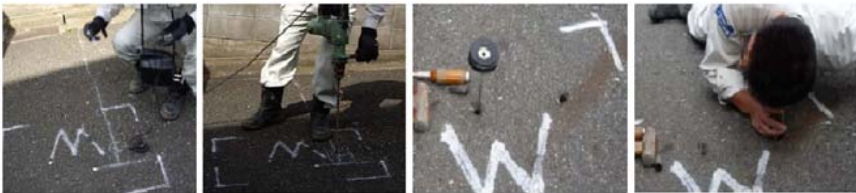
Figure 14: Confirmation of leakage at the opening
