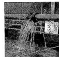
Dia.50mm Falling out of the flange portion Water pressure:2.0 kg/cm 2 , W/Leakage 3.0 m 3 /hrs. Water pressure: 2.5 kg/cm 2 , W/Leakage 3.35 m 3 /hrs Water pressure: 3.0 kg/cm 2 , W/Leakage 3.97 m 3 /hrs
