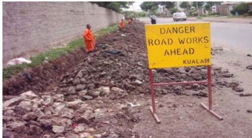
Put warning signs when trenching along road
