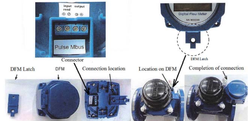
Example of Fixing New DFM for Small size meters
