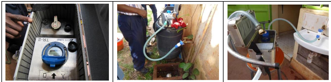
Figure 17 Installation drawing of electronic meter
