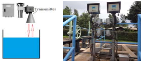
Figure-13 Example of Ultrasonic level meters
