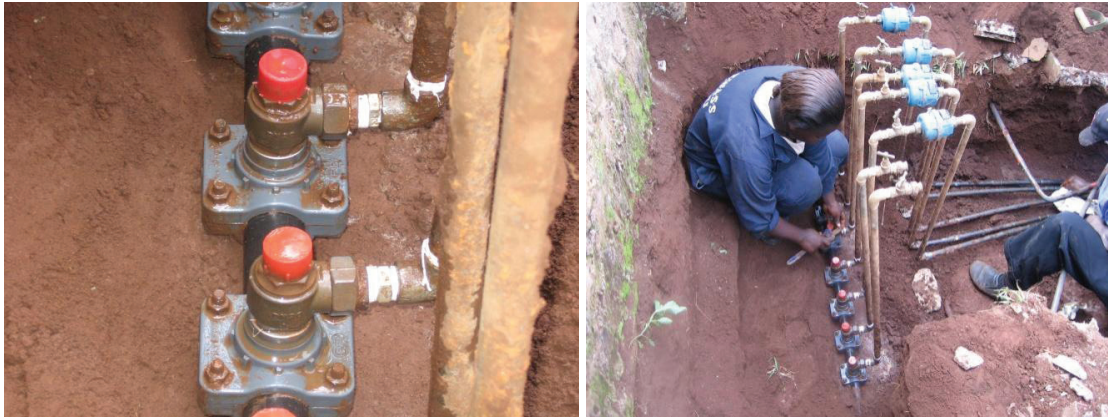
Figure 3.1: Tapping with standardized saddle clamp and ferrule (tap)
