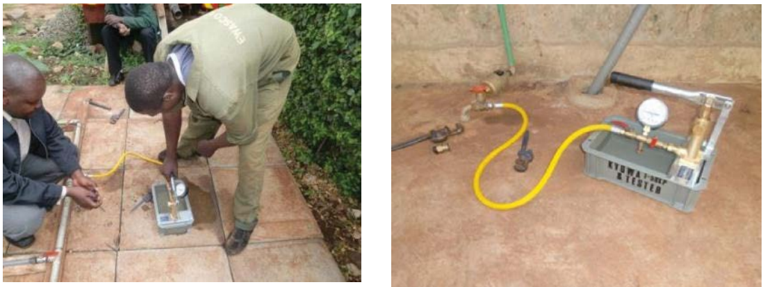
Figure 8.17 Water Pressure Test
