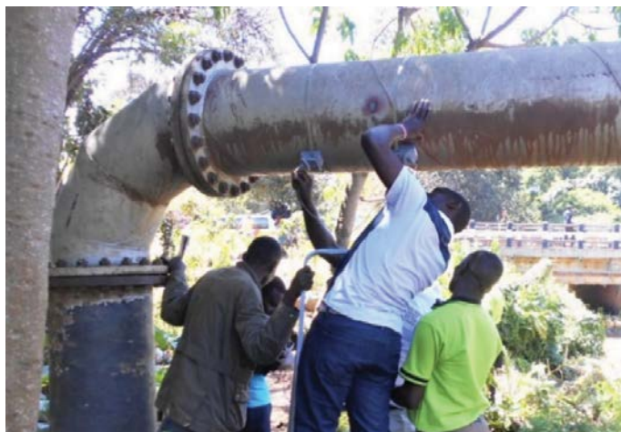
Installing Ultrasonic Flow Meters for measurement (ELDOWAS)
