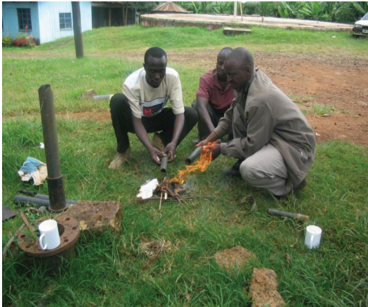
Figure 2.13: Softening Pipe by Heating
