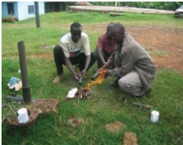
Figure 8.8: Making Fire Coupling (used for pipe connections in Kenya)
