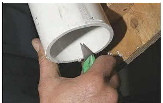
Figure 2.7: Unchamfered dimensions being deburred
