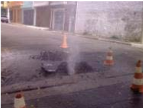
Figure 8.2: Visible Leakage (Surface leakage)
