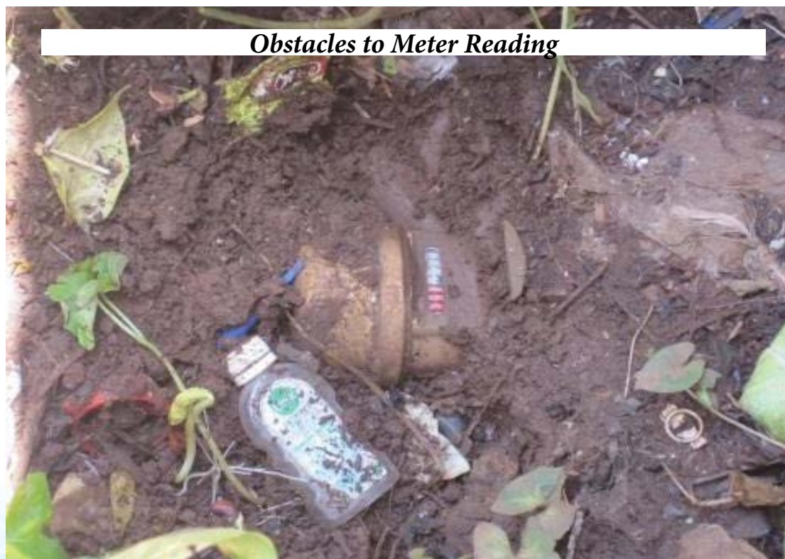
Figure 6.7: Water Meter Covered in Mud
