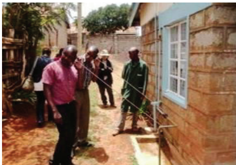
Figure 5.4: Leak detection using listening stick on pipe fittings
