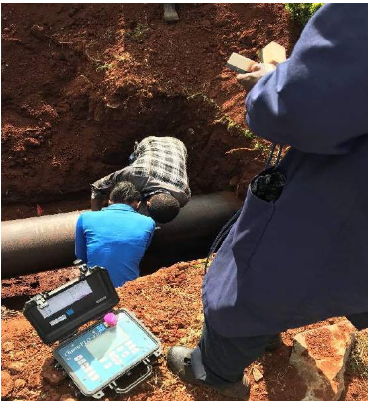
Installation of leakage detection equipment
