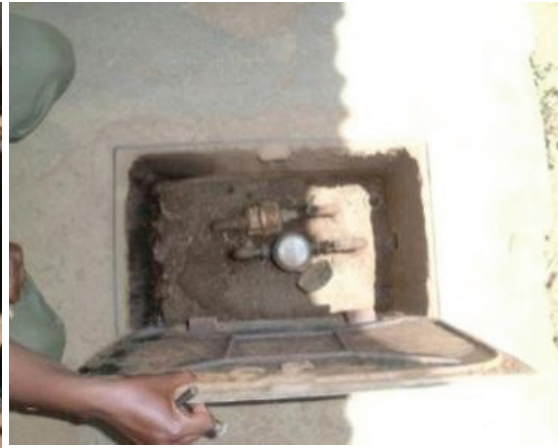
Photo 3.2: Installation of Customer Meters in a meter box
