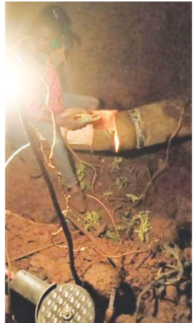
Technician is fixing leakages of pipe at night (MUWASCO)
