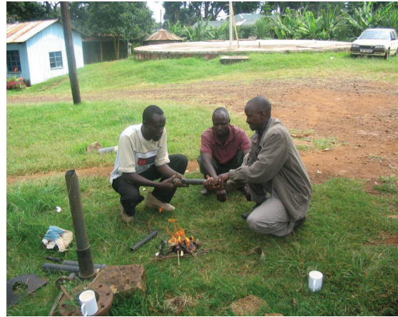
Figure 2.14: Making Fire-made Coupling from Softened Pipes
