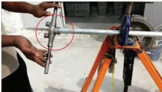
Figure 2.31: Threading of pipe with diestock
