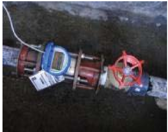
Figure 8.6: Measure the flow volume into the block
