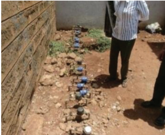
Photo 3.1: Installation of Customer Meters without meter box
