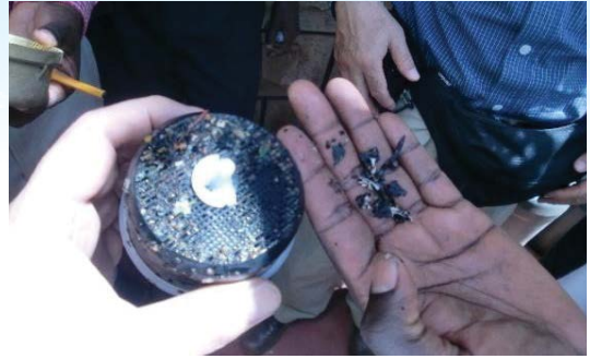
Figure 6.2: Roots at Customer Meter (Embu WSP)
