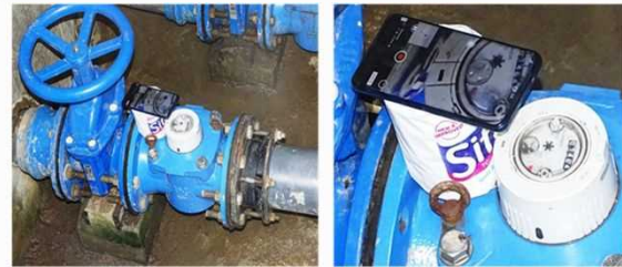
Checking accuracy of bulk meter using smartphone with time stamp camera and potable UFM
