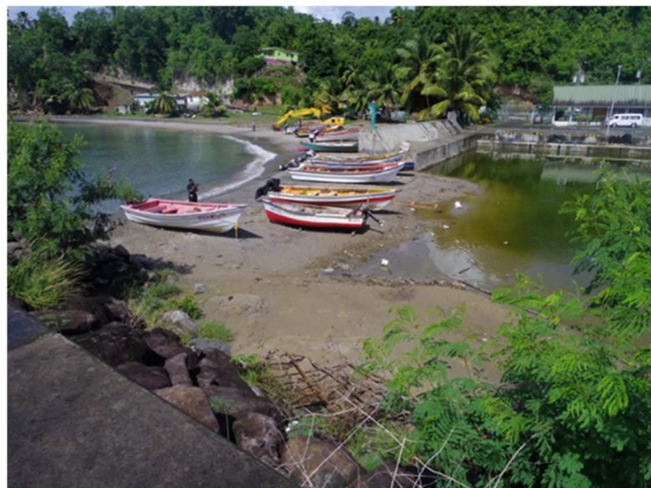
Photo 3-2-1-1 (1) Complete closure of port entrance (November 4 th , 2015)
