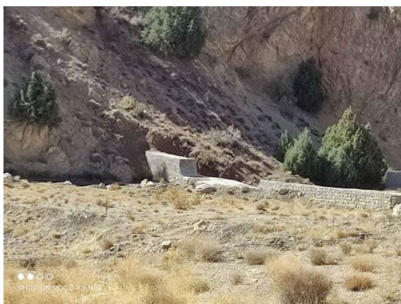
Erosion Control Weirs in the Mountains (Vala Area)
