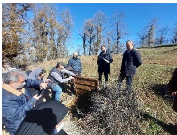
Valve to Regulate Reservoir Distribution (Fazelabad Area)
