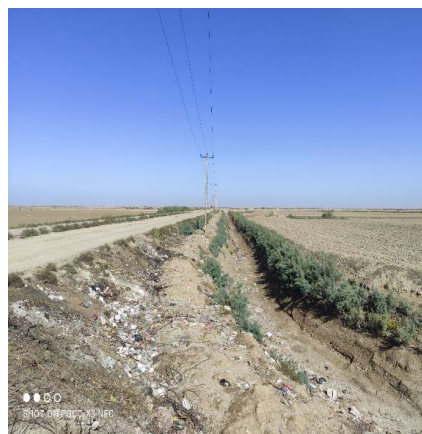
Drainage Canals in Earthen Canals (Sabz Dash Ghaleha Area)
