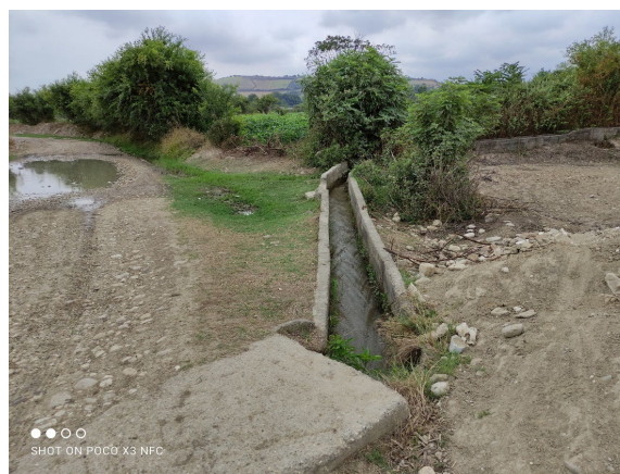
Conduit from the Fixed Weir to the Reservoir (Gerankooch Area)
