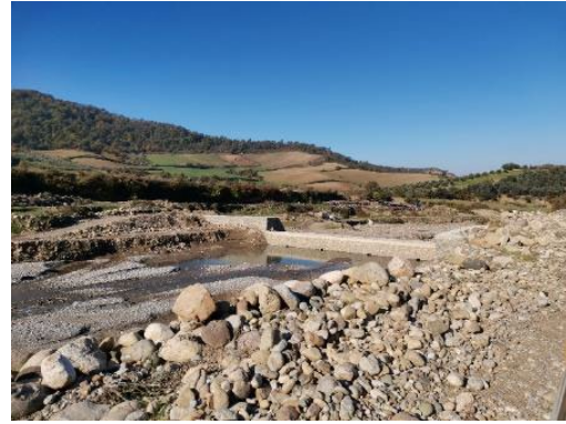
Hilly area: Erosion control weirs in rivers
