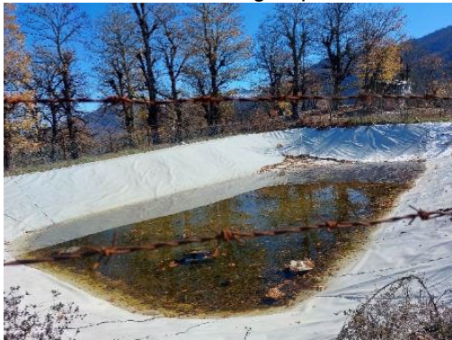
Hilly area: Reservoir maintenance by JAO
