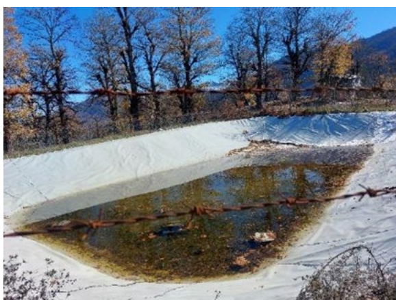
Dug-in Reservoir (Fazelabad Area)
