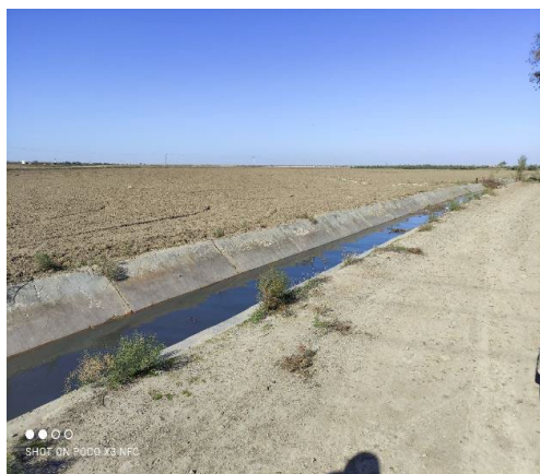
Lining Irrigation Canals (Sabz Dash Ghaleha Area)
