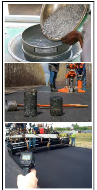
Figure 4-26 Surface test of pavement
