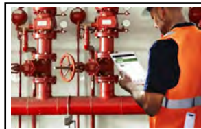
Figure 4-xx Fire safety inspection
