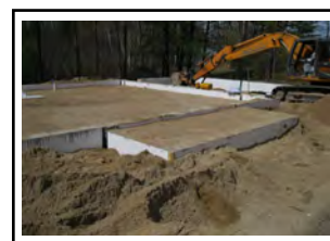
Figure 4-10 Backfilling
