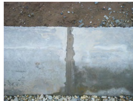
Incomplete process of concrete works
