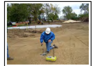
Figure 4-21 Compaction of subbase
