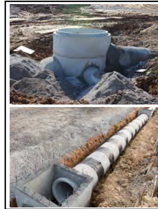
Figure 4-xx Manhole and pipe connection
