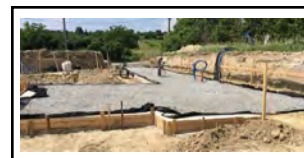
Figure 4-11 Gravel Bedding
