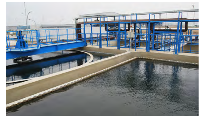
Figure 2-38 Water storage tank
