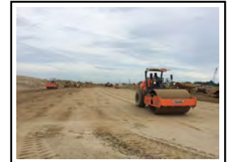
Figure 4-20 Compaction of subgrade
