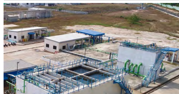
Figure 2-11 Water Purification Plant
