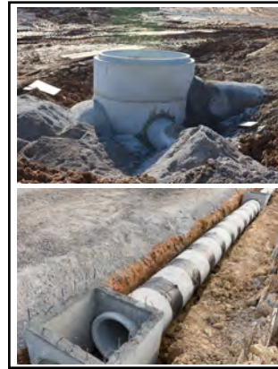
Figure 4-xx Manhole and pipe connection
