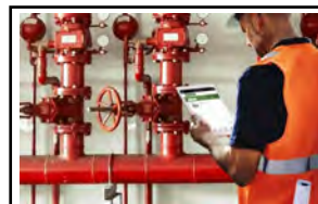
Figure 4-xx Fire safety inspection
