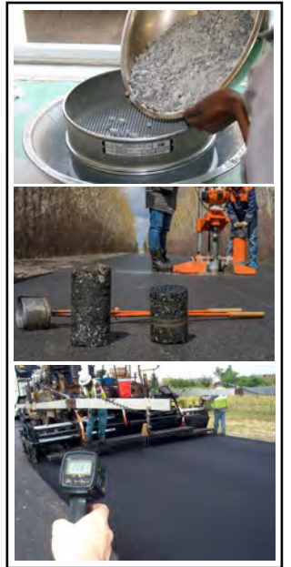
Figure 4-26 Surface test of pavement
