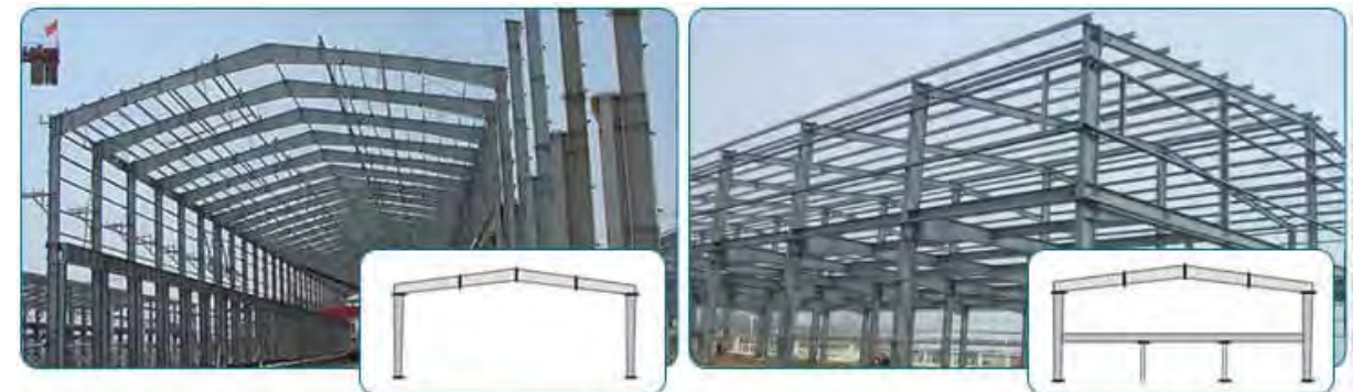
Figure 3-9 Sample of building structures
