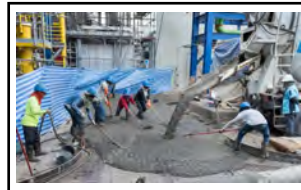
Figure 4-28 Concrete placement
