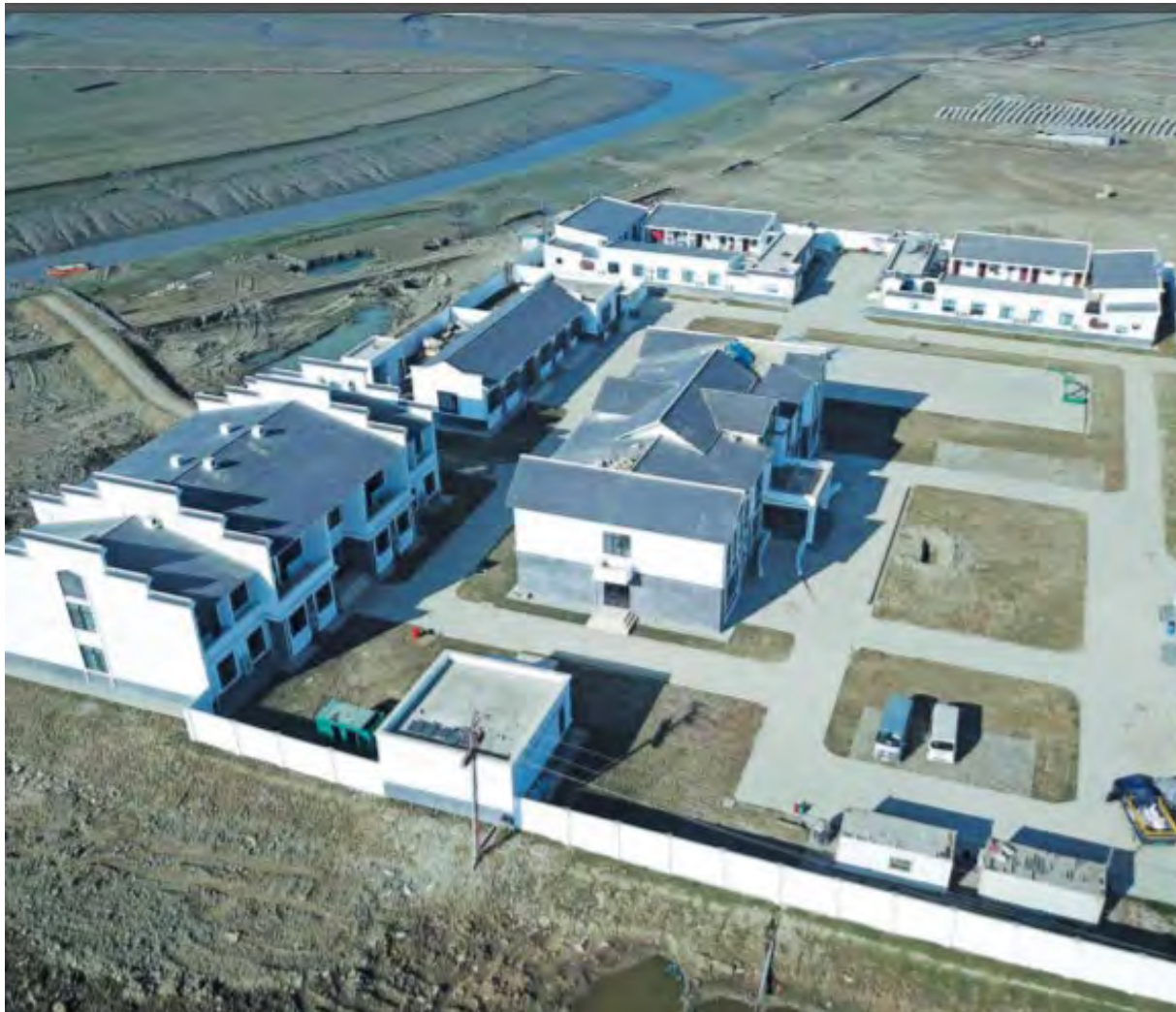
Figure 1-3: Management building of EZ, BSMSN
