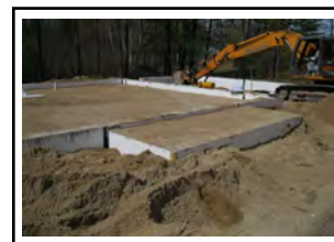
Figure 4-10 Backfilling
