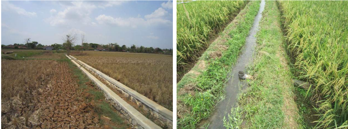
Photo Left: A Typical Lined Tertiary Canal (Central Java), Photo Right: A Typical Earthen Tertiary Canal (West Java)
