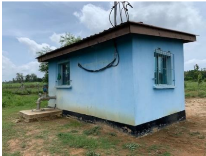
Exterior of Borehole (New Borehole)
