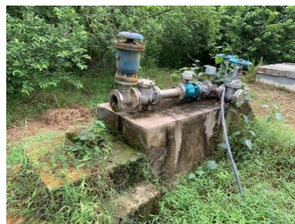
Borehole with Pump Removed (Rehabilitated Borehole)
