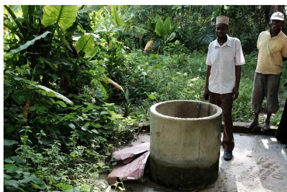
Photo 2.8 Artesian Borehole in Kianga Scheme
