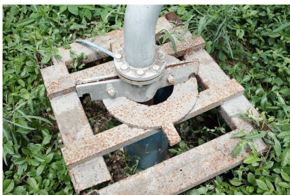
Photo 2.6 Borehole in the Factory
