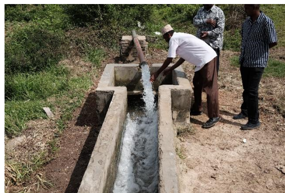
Photo 2.11 Irrigation Canal in Bumbwisudi
