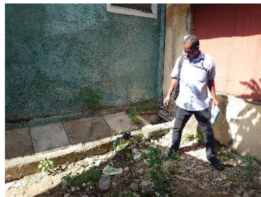
Meter installation status
