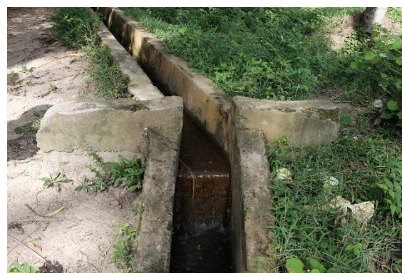
Photo 2.9 Irrigation Canal of Kianga Scheme
