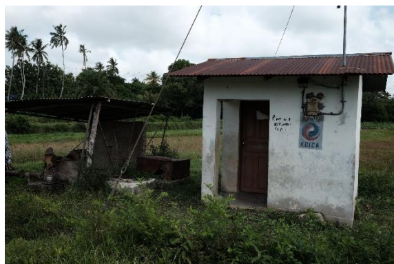
Photo 2.10 Borehole in Bumbwisudi Scheme
