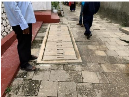
Manifold in Stone Town
