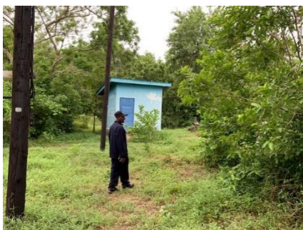
Borehole with Pump Removed (Rehabilitated Borehole)
