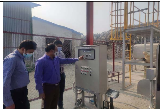
Confirmation of status of incinerator operation and maintenance by the Department of Environment (March 2022)
