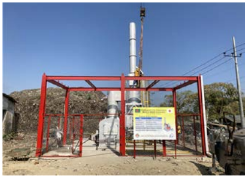
Installation of the small medical waste incinerator (January 2022)
