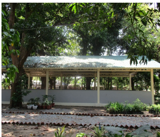
Newly constructed workshop shed among standing trees
