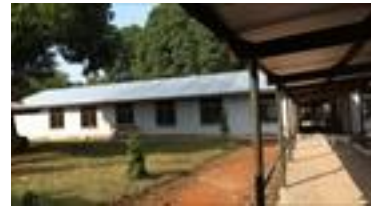
Accommodation facility under renovation
