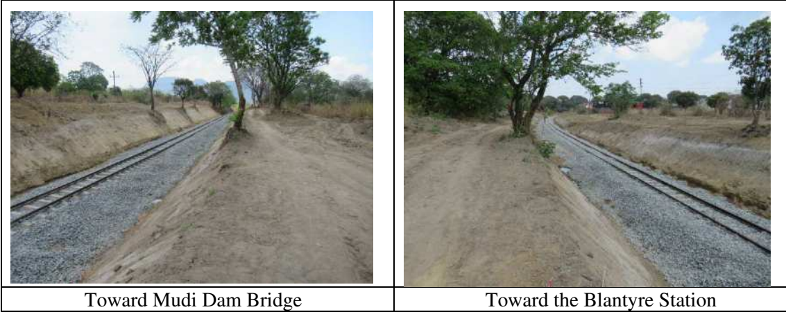
Figure 3-4.20 Situations after Railway Track Elevation Lowering Works (As of September, 2021)
