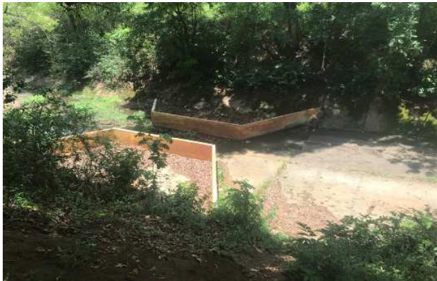
Monitoring Facilities at the Spillway of Mudi Dam
