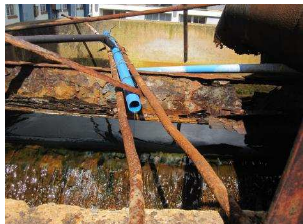
Figure 3-3.4 Dosing Coagulant
