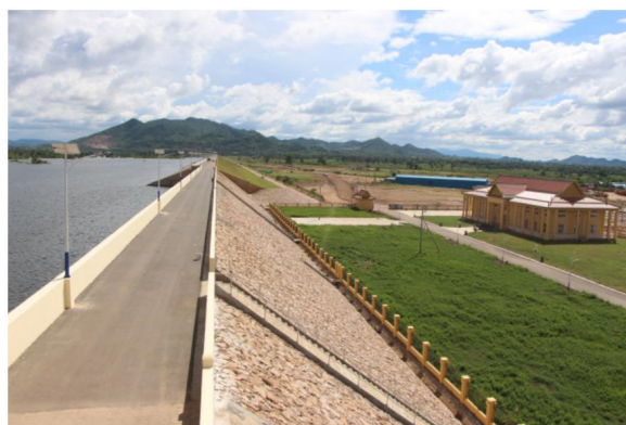
Road on the crest of Left Bank Earth Dam and Concrete Face Rockfill Dam
