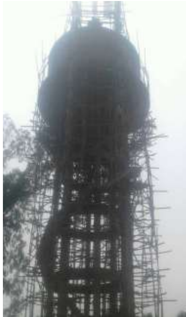
Over Head Tank 225 cum is under construction. Project-3
