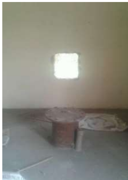
Under construction of Deeptube well at Auraha Tole. Project 3
