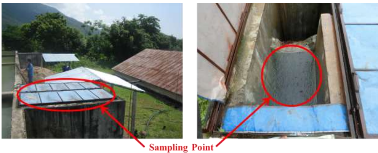
Photo-4. Sampling Points in Outlet of Slow Sand Filter
