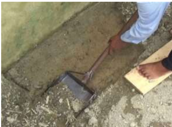
Photo 2.20 Scraping Surface Sand
