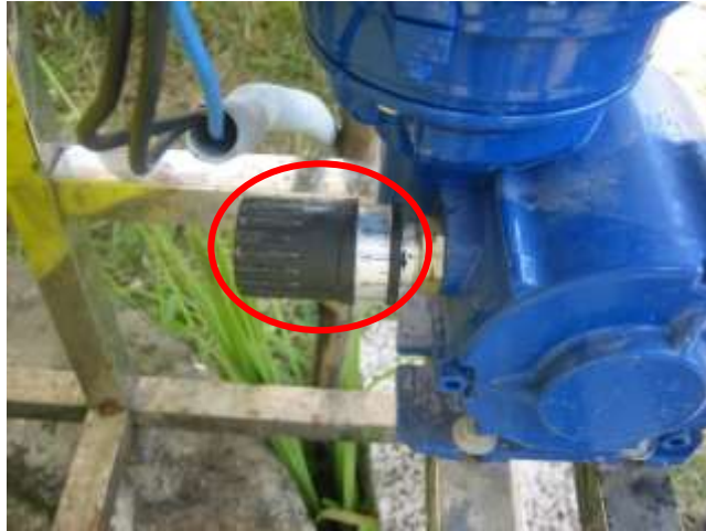
Photo 2.34 The Location of Stroke Adjusting Screw
