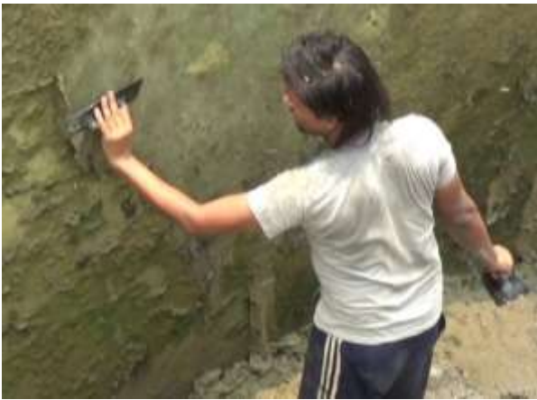
Photo 2.6 Cleaning of Wall
