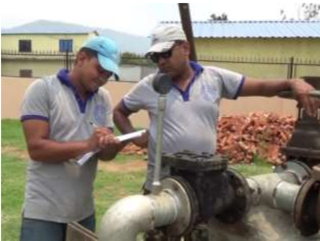
Photo-1. Checking Pressure Gauge
