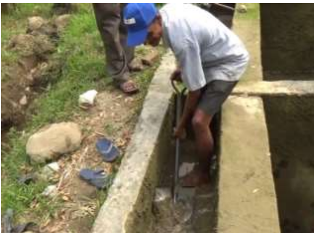
Photo-3. Cleaning of Inlet Chamber
