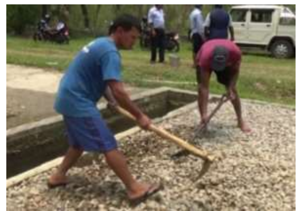
Photo 2.13 Backfilling the Washed Gravel
