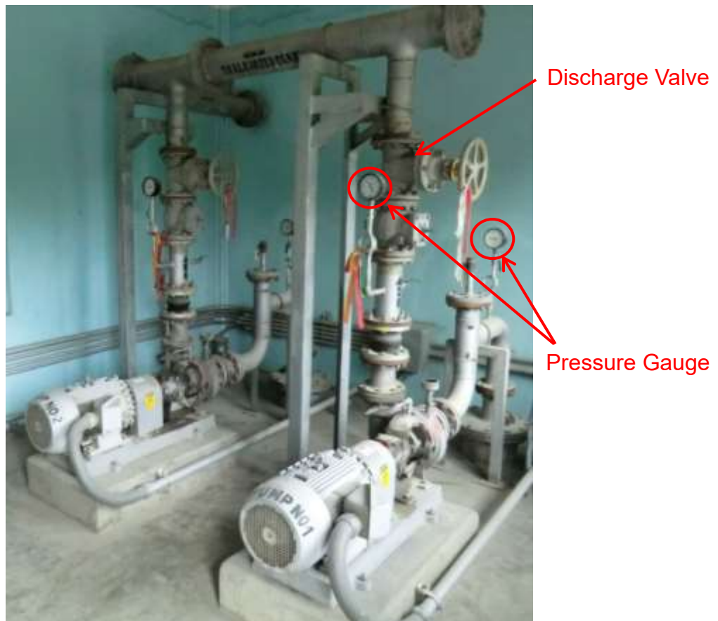
Photo-1. Typical System of Volute Pump
