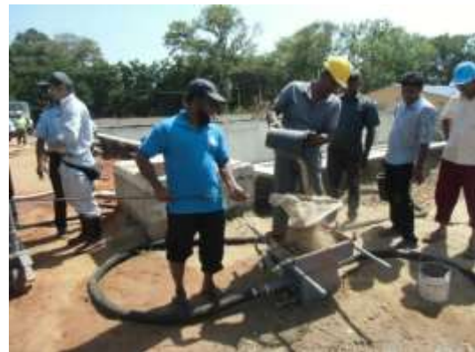
(6) Putting used sand into feeder
