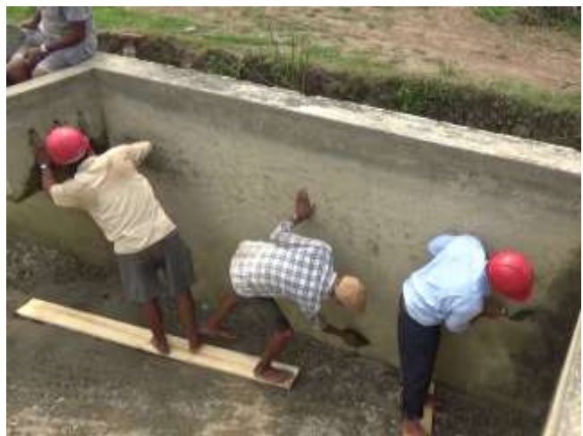
Photo-2. Cleaning Inside Walls
