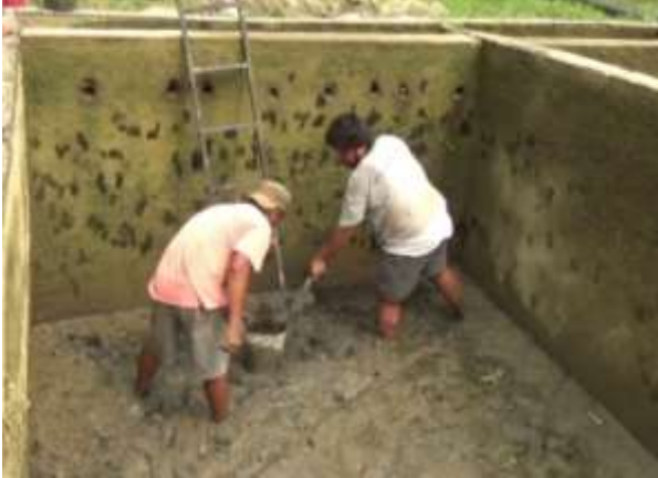
Photo 2.4 Removing Settled Sludge
