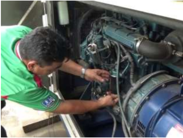
Photo-1. Checking Loose Fastenings
