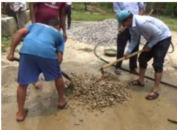
Photo 2.12 Washing Gravel with Clean Water
