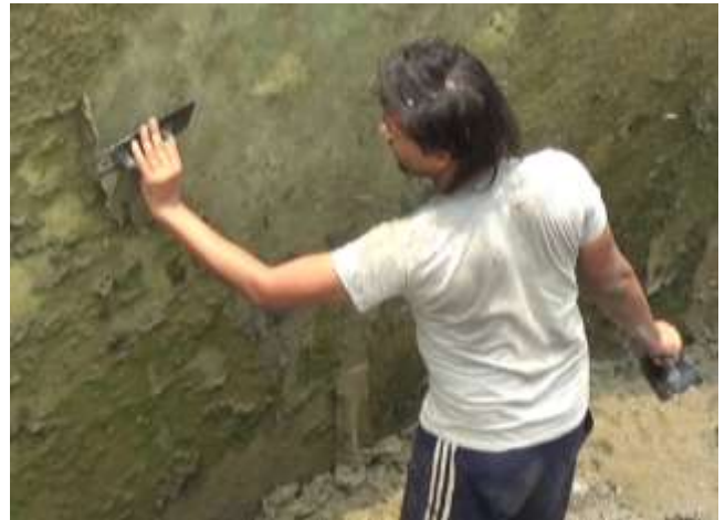
Photo-4. Cleaning of Wall
