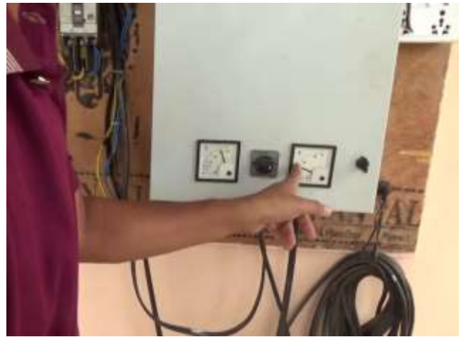
Photo-2. Checking Ampere
