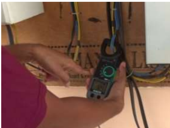
Photo 2.7. Measuring Ampere
