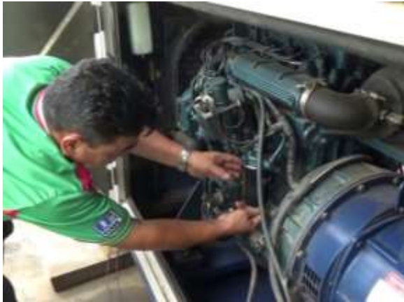
Photo 2.9 Checking Loose Fastenings
