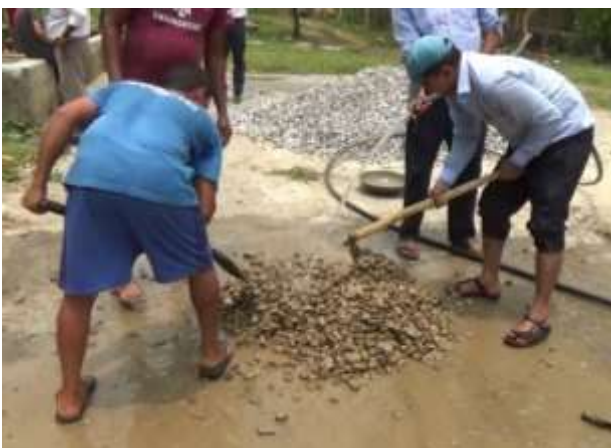
Photo-3. Washing Gravel with Clean Water
