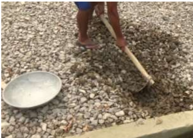
Photo-1. Excavating Gravel
