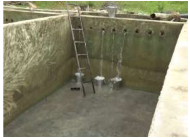
Photo 2.7 Cleaning of Bottom with Water
