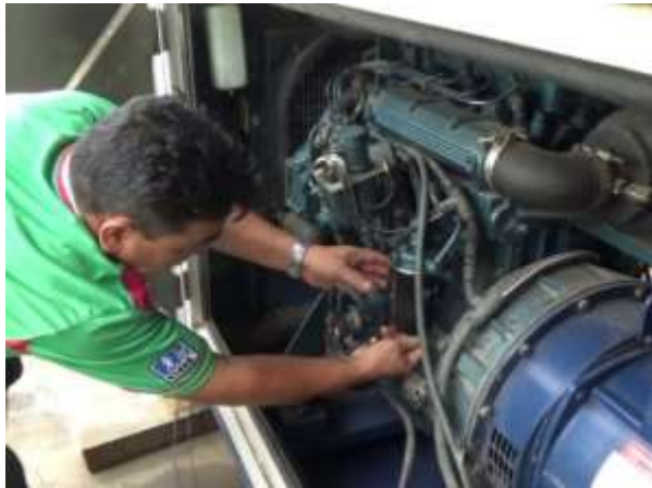
Photo 2.44 Checking Loose Fastenings
