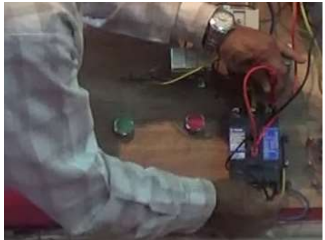
Photo-4. Checking Continuity
