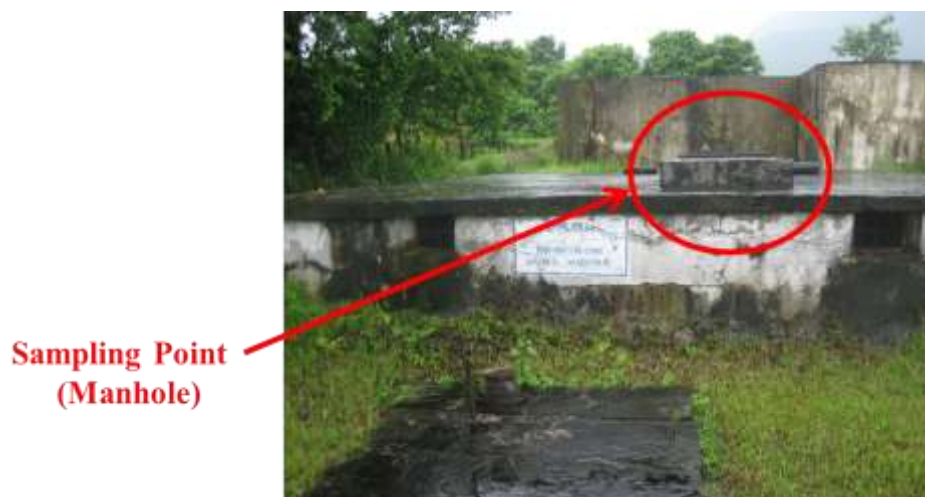
Photo-5. Sampling Point in Clear Water Reservoir
