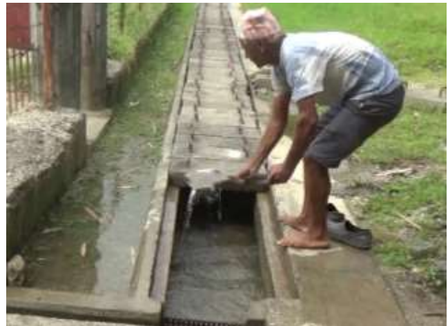
Photo-2. Removing Sediments
