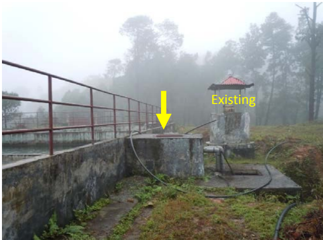
Photo-12 Chautara WUSC on September 11, 2016 Chlorine is injected on the top of the chamber. (red arrow)
