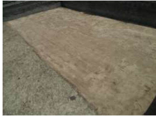
(4) Completion of Scraping Filter Sand
