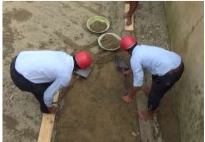
Photo-3. Scraping Surface Sand
