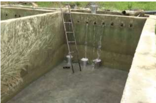
Photo-5. Cleaning of Bottom with Water
