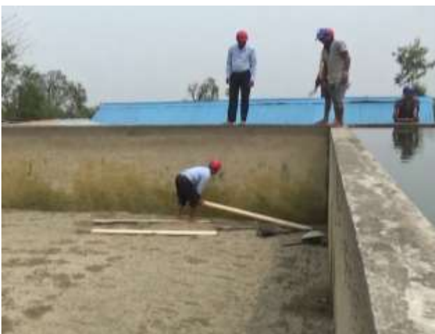
Photo-1. Preparation of Stage Planks
