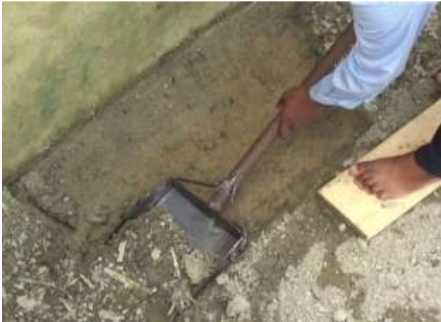
Photo-3. Scraping Surface Sand
