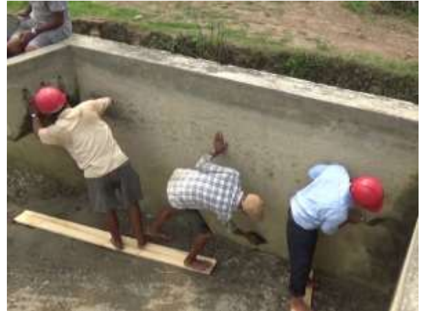
Photo 2.19 Cleaning Inside Walls
