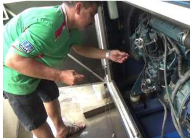
Photo-2. Checking Level of Engine Oil
