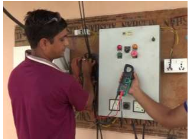
Photo-2. Measuring Voltage
