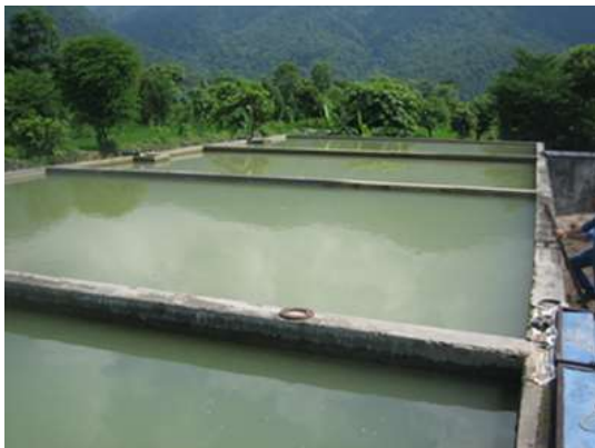
Photo 1.2 Outline of Roughing Filter (Left: Pragatinagar WUSC, Right: Beljhundi WUSC)
