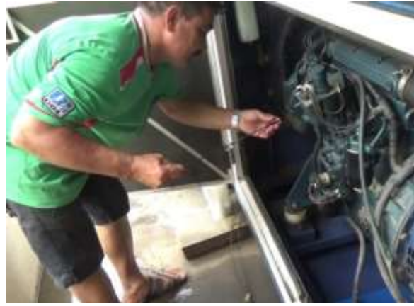
Photo 2.10 Checking Level of Engine Oil
