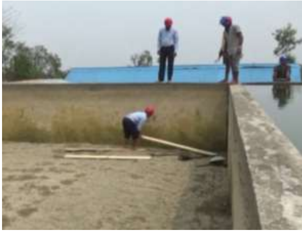
Photo 2.18 Preparation of Stage Planks
