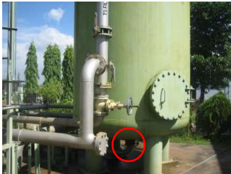
Photo 2. Sampling Point of Pressure Filter
