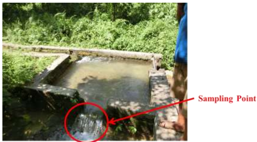
Photo-1. Sampling Point in Outlet of Intake Facility
