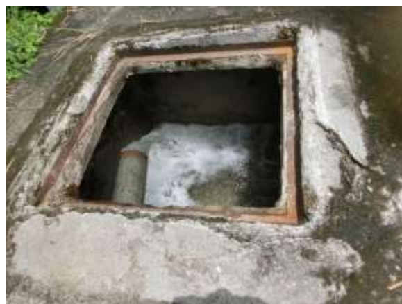
Photo 1.1 Rectangular Receiving Well (Left, Dhulabari WUSC), Ground Type Collection Chamber (Right, Besisahar WUSC)
