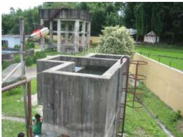
Photo 1.1 Rectangular Receiving Well (Left, Dhulabari WUSC), Ground Type Collection Chamber (Right, Besisahar WUSC)
