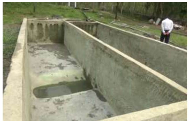
Photo-6. Completion of Cleaning
