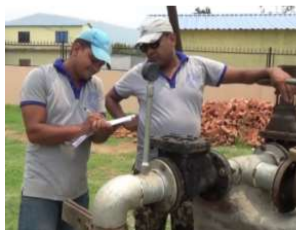
Photo 2.39 Checking Pressure Gauge
