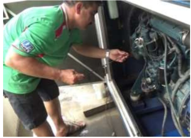
Photo 2.45 Checking Level of Engine Oil
