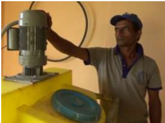
Photo-1. Daily Inspection of Mixer
