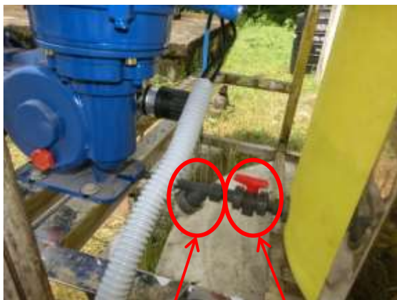
Photo 2.33 The Location of Strainer, Suction Valve and Pressure Gauge
