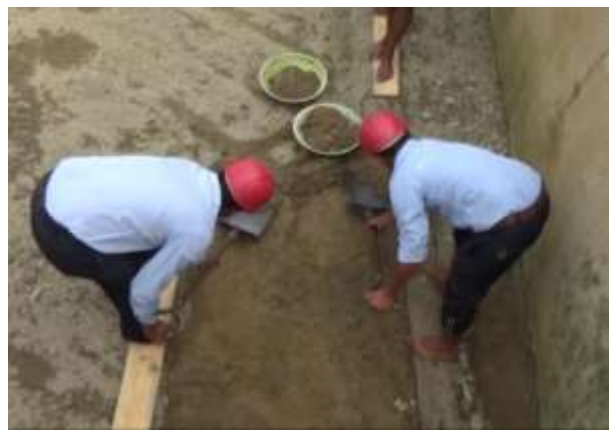
Photo 2.20 Scraping Surface Sand
