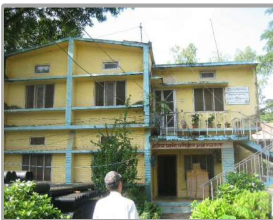
Photo 1: Full view of building
