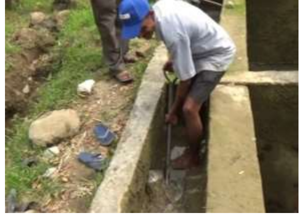
Photo 2.5 Cleaning of Inlet Chamber
