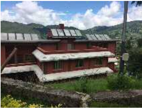
【Photo 8】 Accommodation building B
