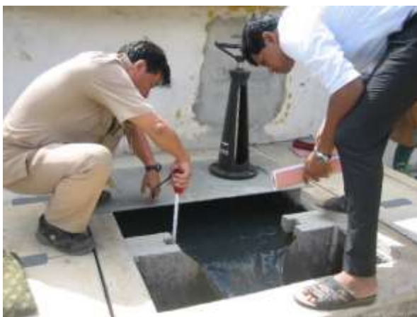
Photo 2.16 Measurement of Filtration Rate at V-notch
