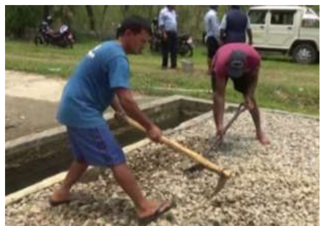
Photo-4. Backfilling the Washed Gravel
