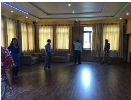
【Photo 15】 Recreation Room (Museum Building)
