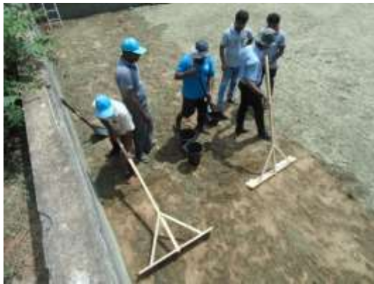
(3) Scraping dried Filter Sand
