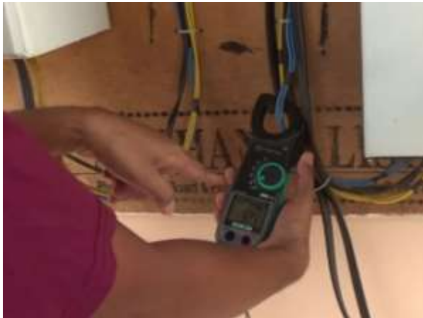
Photo 2.42 Measuring Ampere
