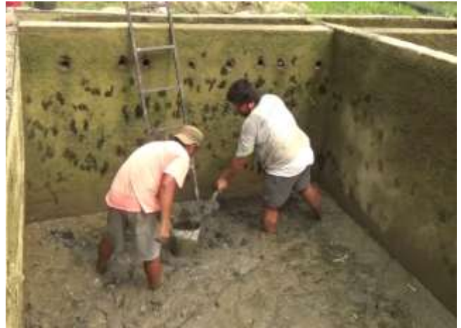
Photo-2. Removing Settled Sludge
