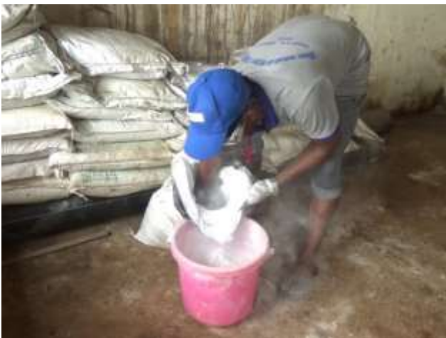
Photo-2. Measuring the Required Amount of Bleaching Powder
