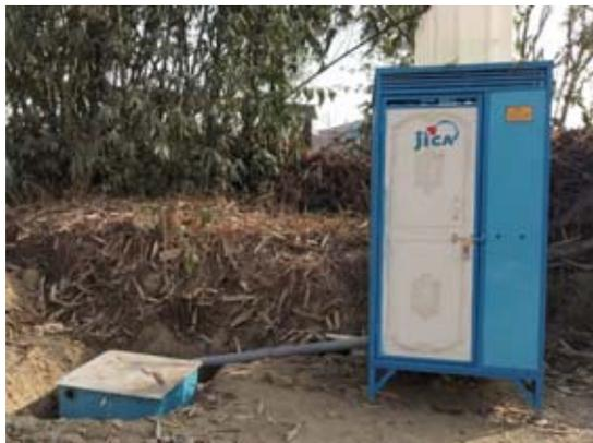
Figure 2.11 Installation of the temporary toilet
