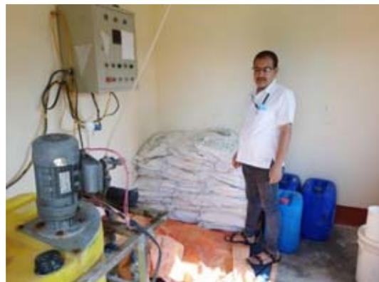
Figure 2.12 Chlorine Injection Unit and Bleaching Powder
