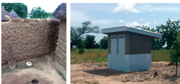
Left: Traditional latrine in the Far North Region. Right: Ventilated Improved Pit (VIP) latrines built for project to improve sanitation in the Far North Region. (Photos: Miguel Vargas-Ramirez, World Bank)
