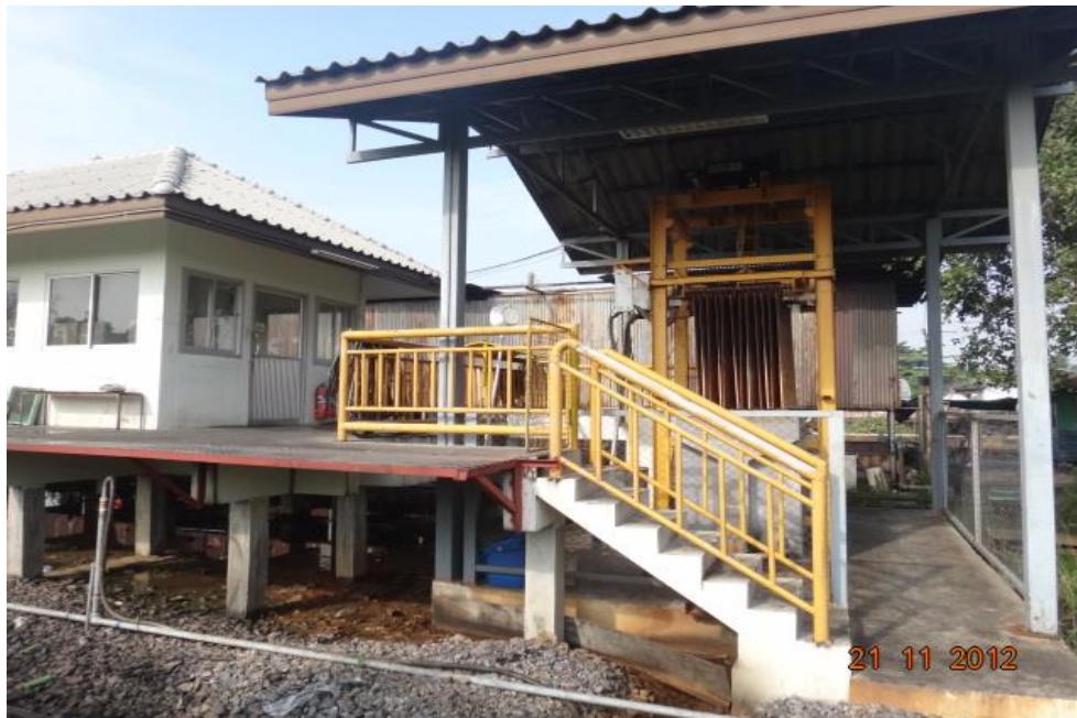
Photo. 2.4-17 Load Test Area
