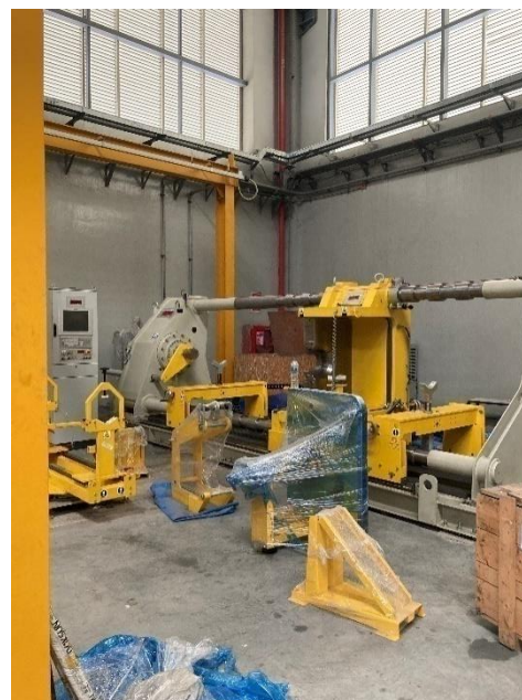
Photo. 2.4-4 Heavy maintenance Area2
