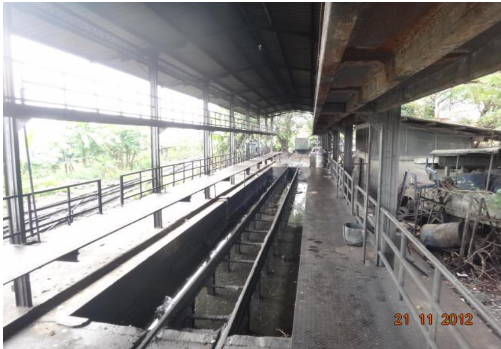
Photo. 2.4-18 Locomotives Washing Area
