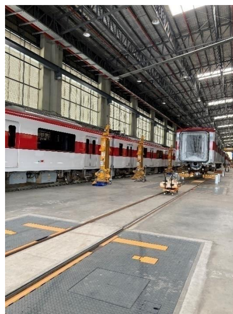
Photo. 2.4-2 Red Line Repair Line
