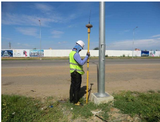
Survey on Road
