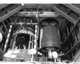
Construction situation line 2
