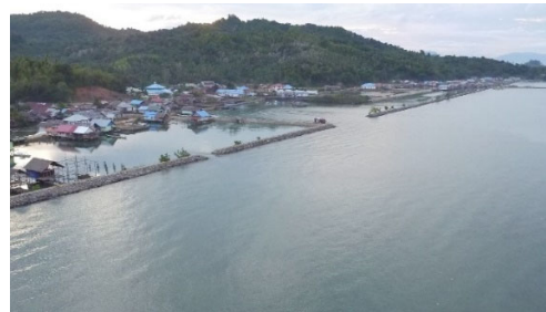
Figure 4-82 Breakwater with cobble stones Pantai Tanjung Bunga, Kabupaten Konawe Utara
