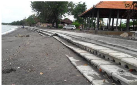
Figure 4-83 Concrete Steps Revetment 134 Desa TukadMungga, Bali North
