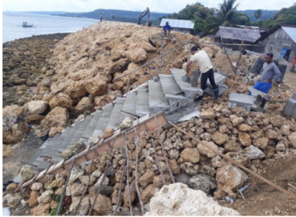
Figure 4-85 Cobble Stones Revetment 136 Morotai Is., North Maluku
