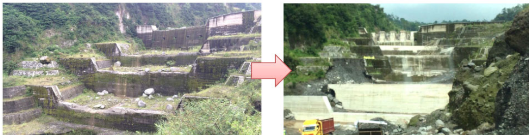
Figure 4-120 Construction Example of Open Type SABO Dam
