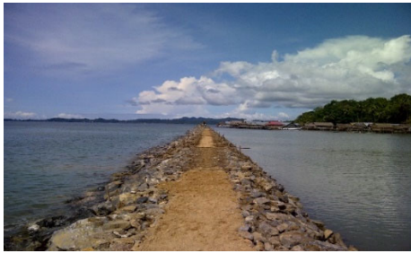
Figure 4-82 Breakwater with cobble stones Pantai Tanjung Bunga, Kabupaten Konawe Utara
