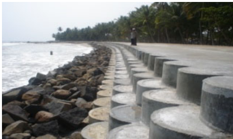
Figure 4-87 Concrete Beach Embankment Pantai Wameo, Kabupaten Bau-Bau, PUPR
