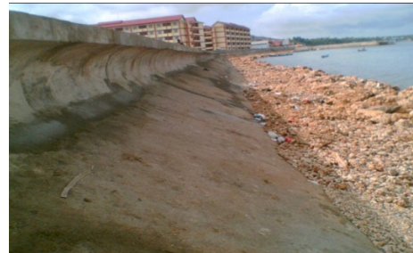
Figure 4-88 Concrete Blocks Revetment Pantai Banding BBWS Mesuji Sekampung
