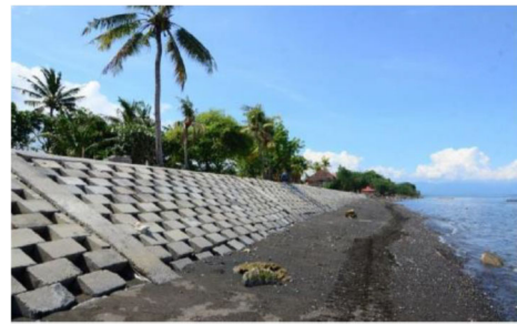
Figure 4-84 Concret Blocks Revetment 135 Desa TukadMungga, Bali North
