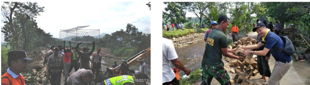
Figure 3-9 Residents in Klaten repair river embankments
