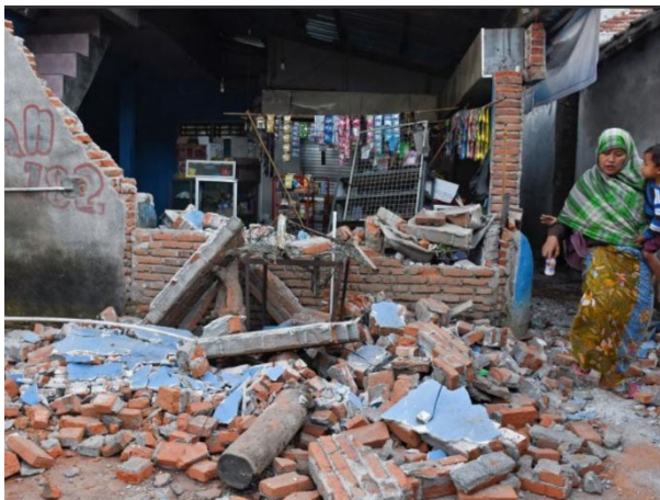
Figure 2-14 Collapsed house due to poor construction methods (1)
