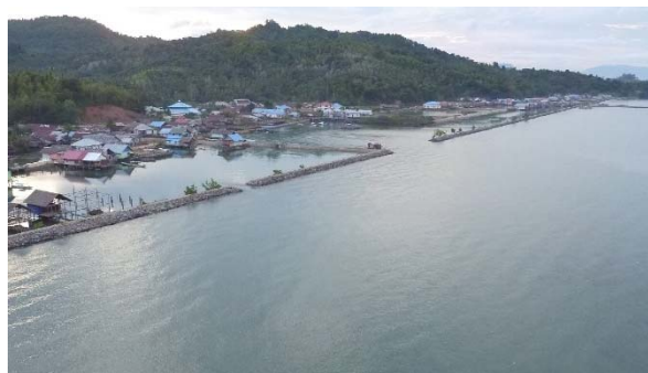
図 4-86 Breakwater with cobble stones 防波堤
