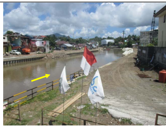
JICA Loan Works ,Downstream of Mahakam Br.
