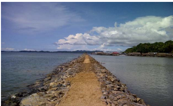
図 4-86 Breakwater with cobble stones 防波堤
