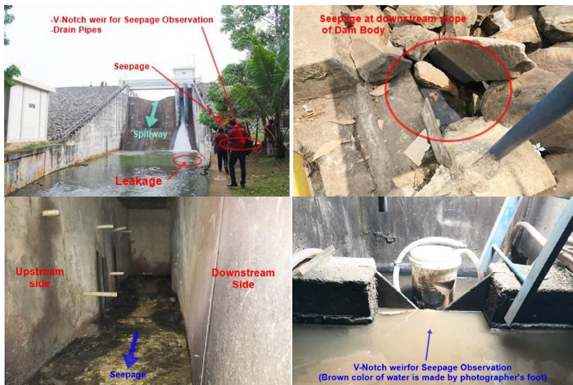
Photo 2.1.3 Situation of Situ Gintung, especially leakage and seepage
