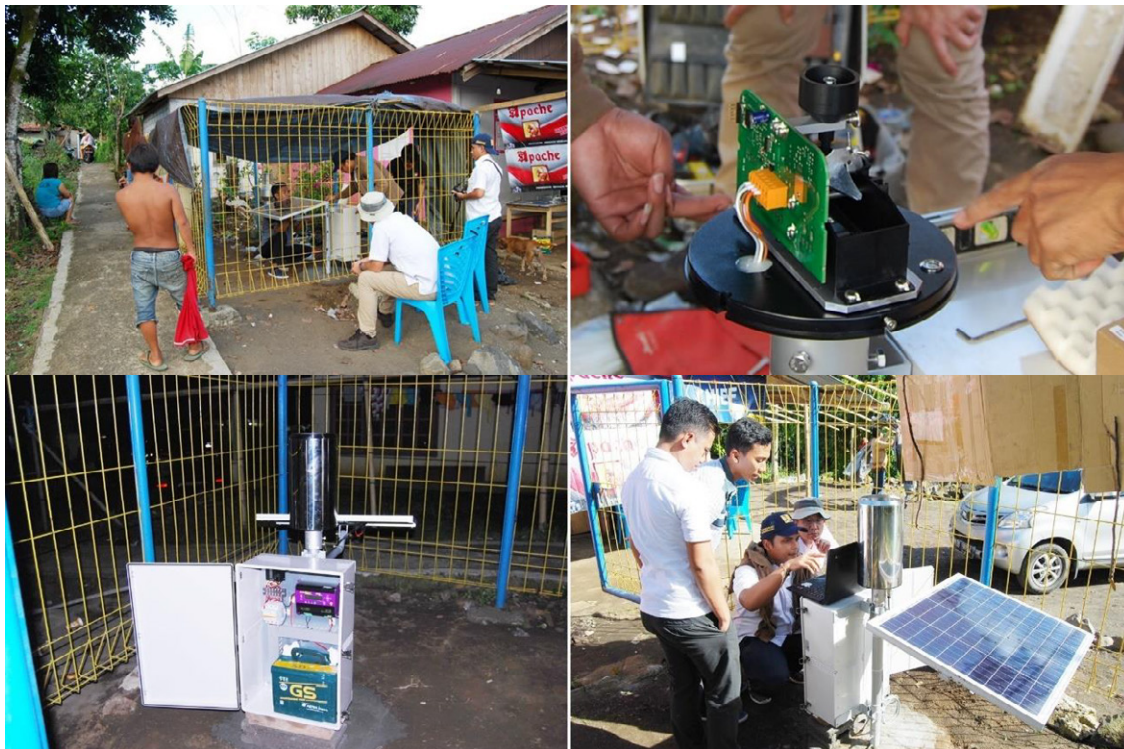
Photo 2.1.10 Installation of ARR at Kuwil Kaleosan with BWS Sulawesi 1
