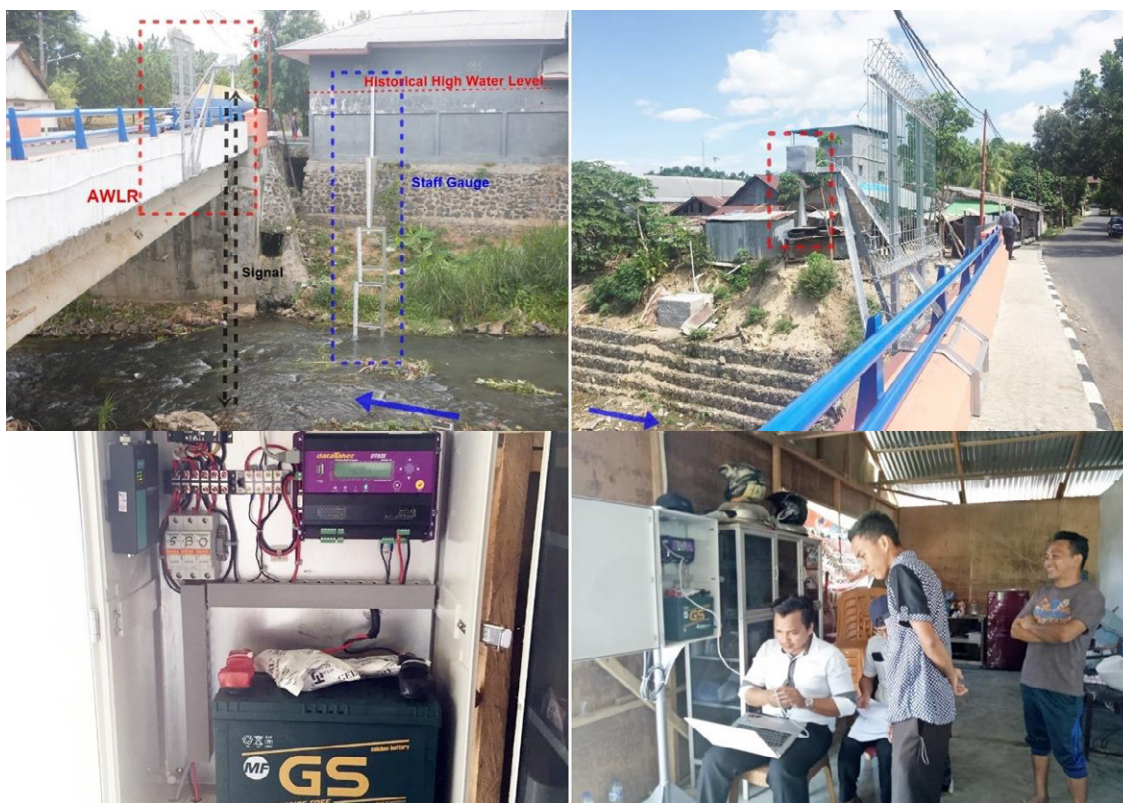
Photo 2.1.11 Installation of AWLR at Tikala with BWS Sulawesi 1
